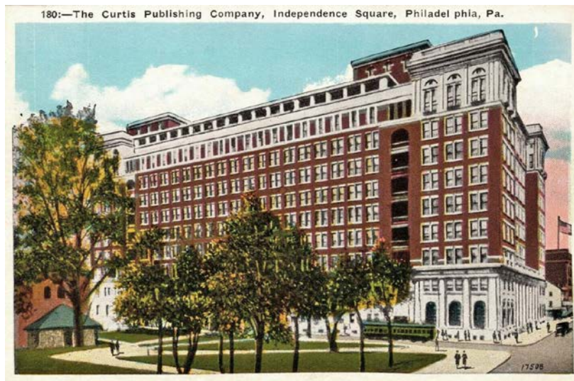
Figure 4 – Curtis Publishing Company Building, designed by Edgar V. Seeler and Spencer Roberts and built in 1907, extant.
