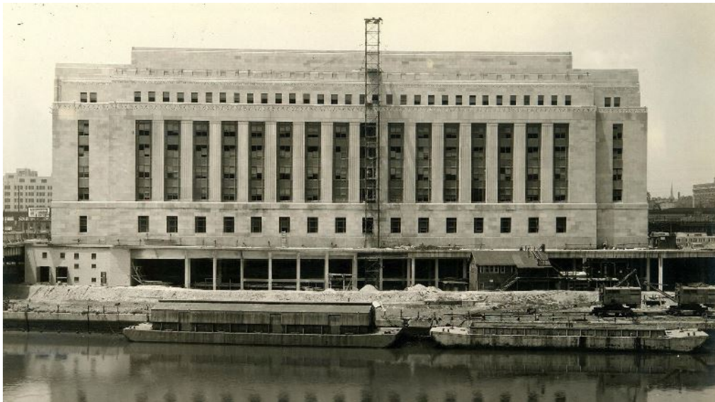
Figure 17 – The U.S. Post office at 30th and Market Streets, designed by Rankin & Kellogg and built in 1931-35 (Athenaeum of Philadelphia).
