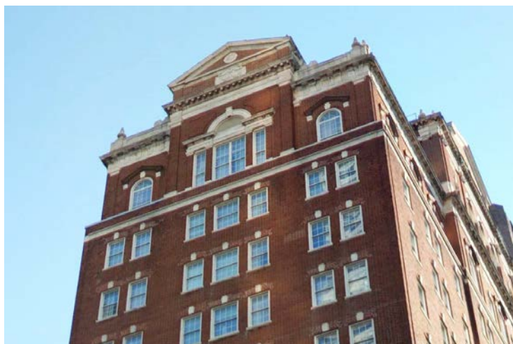
Photo 3 – North elevation, showing the uppermost stories.
