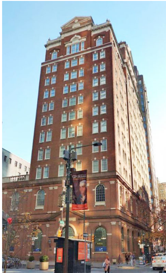
Photo 1 – North and west elevations, looking southeast from 17th and Chestnut.
