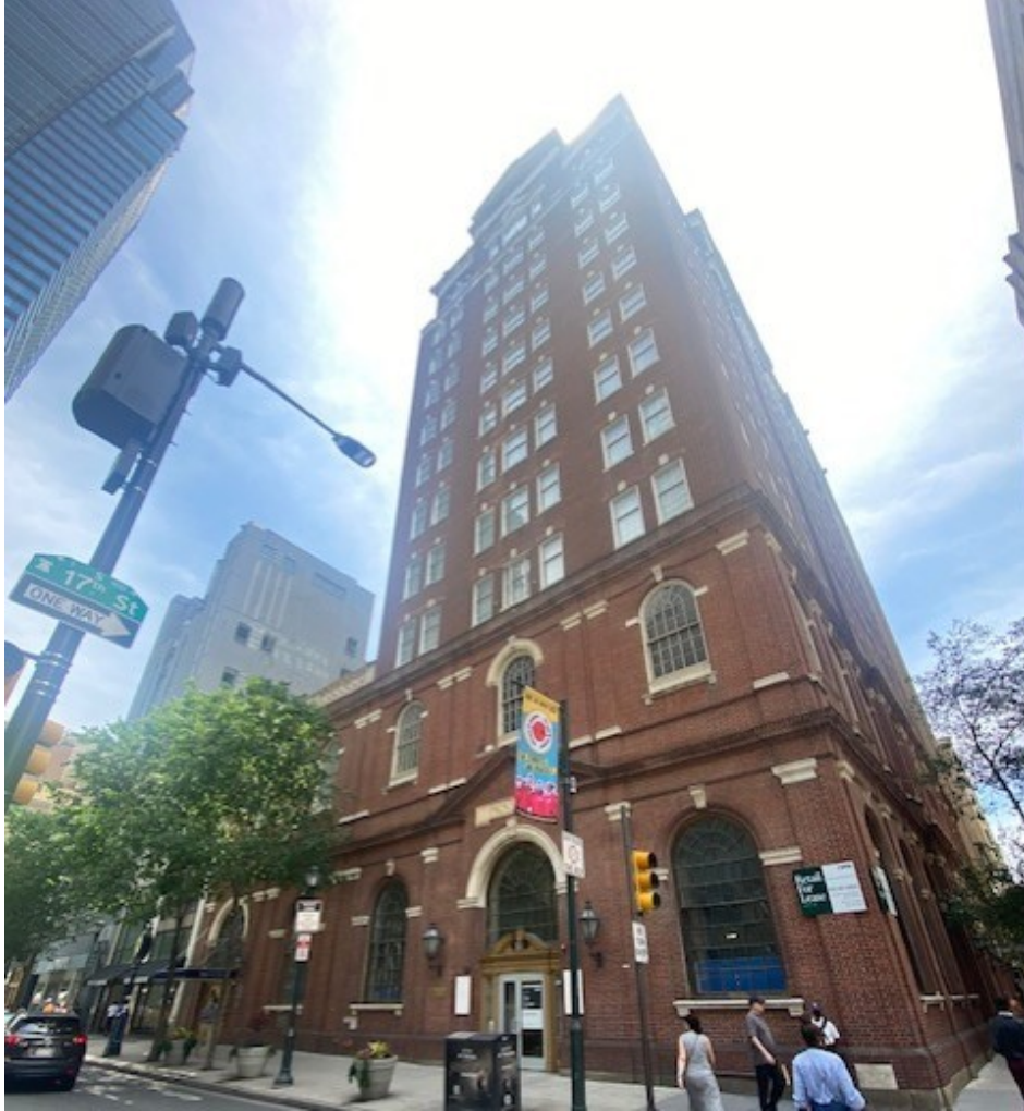
Figure 1: View of the building from Chestnut Street.
