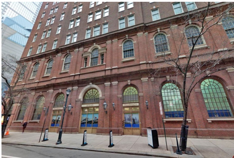
Photo 4 – West elevation, showing the lower stories.
