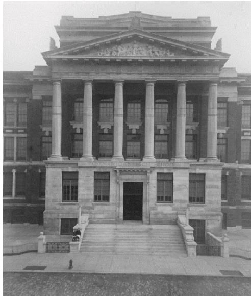
Figure 5 – Germantown High School, designed by Henry DeCoursey Richards and built in 1914-15, extant (Historic Germantown).
