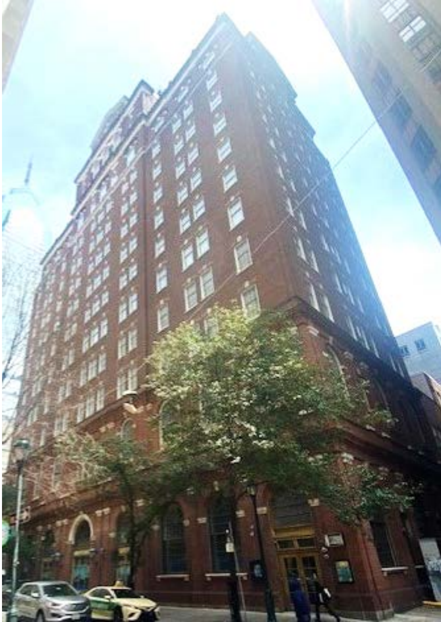
Figure 2: View of building from 17 th Street.
