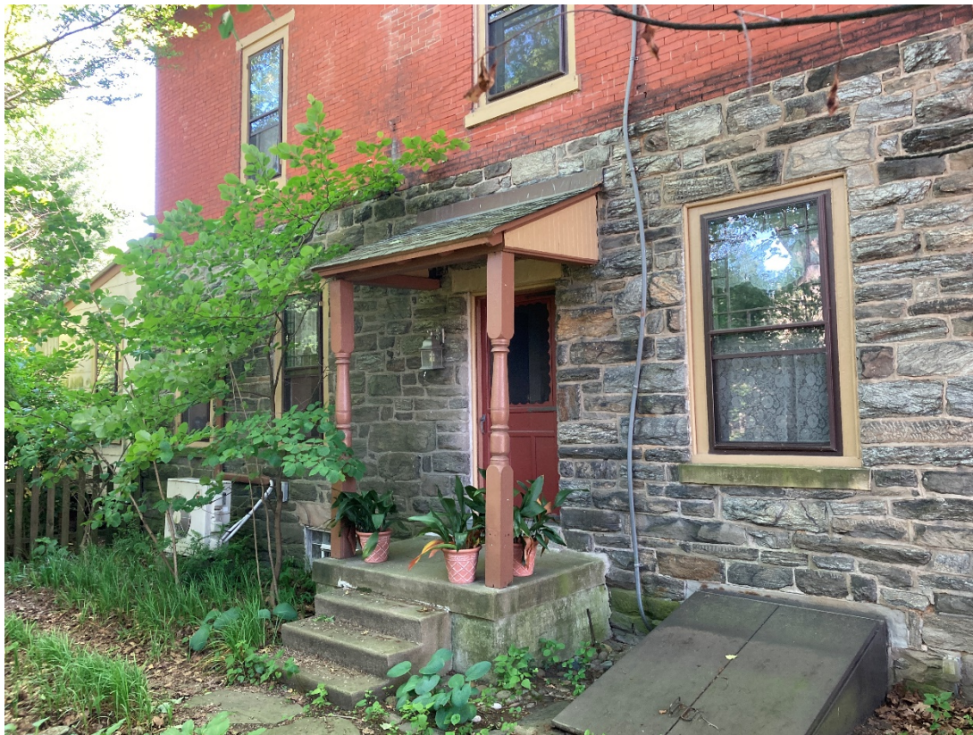
Figure 4: Portion of north façade of 40 W Tulpehocken Street, May 2024. Source: Author
