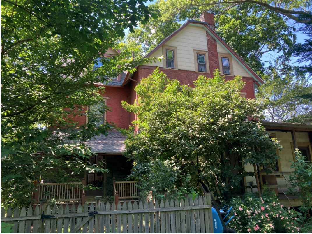
Figure 5: Portion of east façade of 40 W Tulpehocken Street, May 2024. Source: Author
