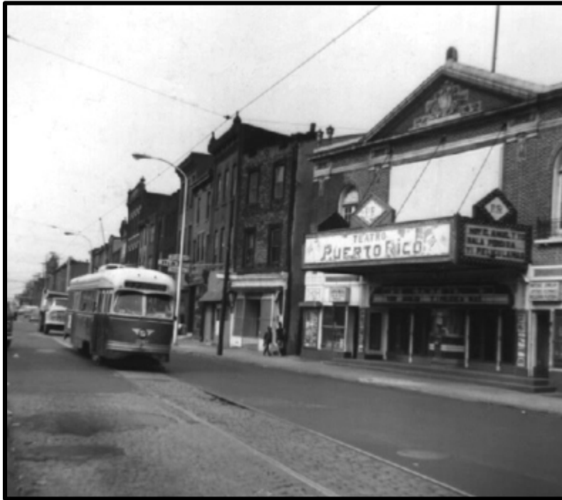
Figure 13. A view of Germantown Avenue with the subject building on right, when it was known as the Teatro Puerto Rico. Source: Cinema Treasures.
