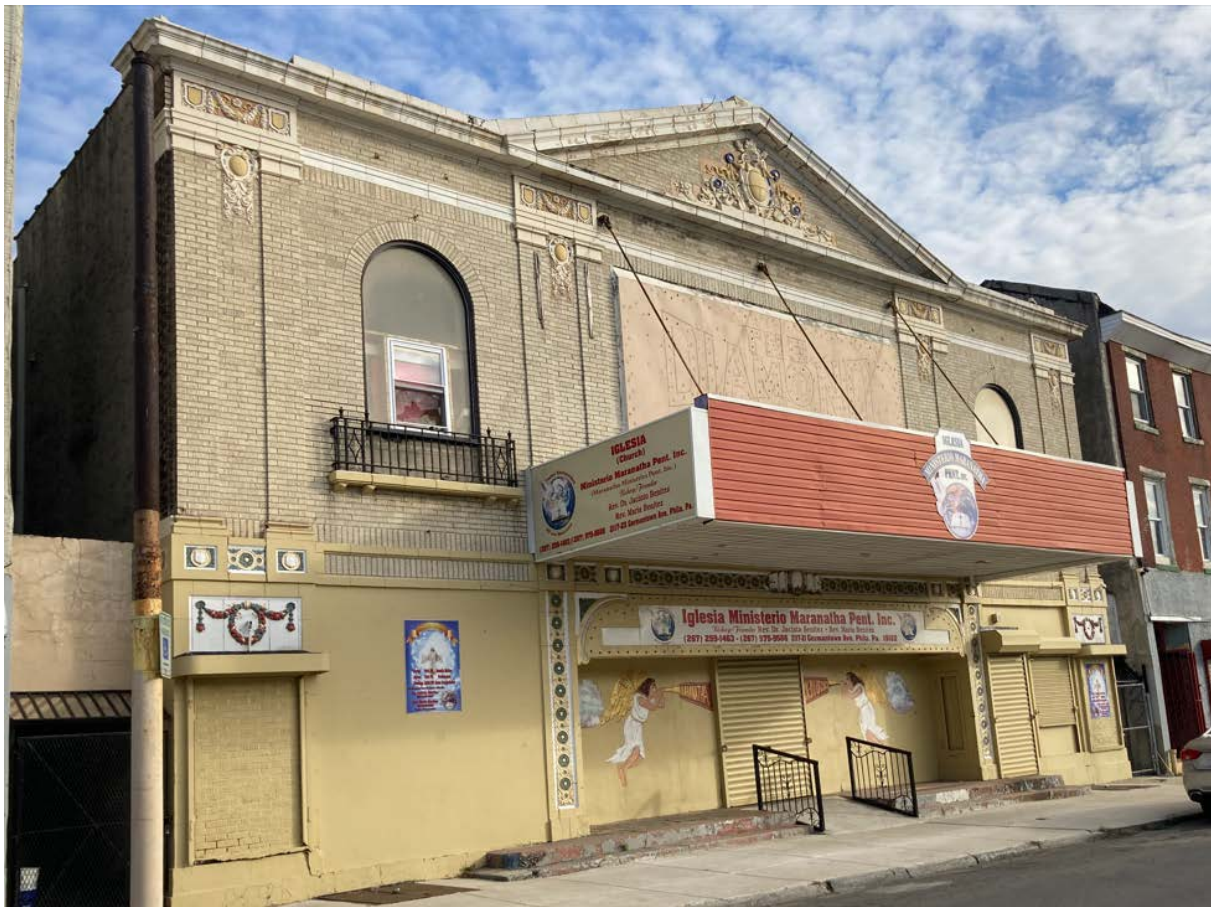
Figure 1: Photo of subject property from the nomination.
