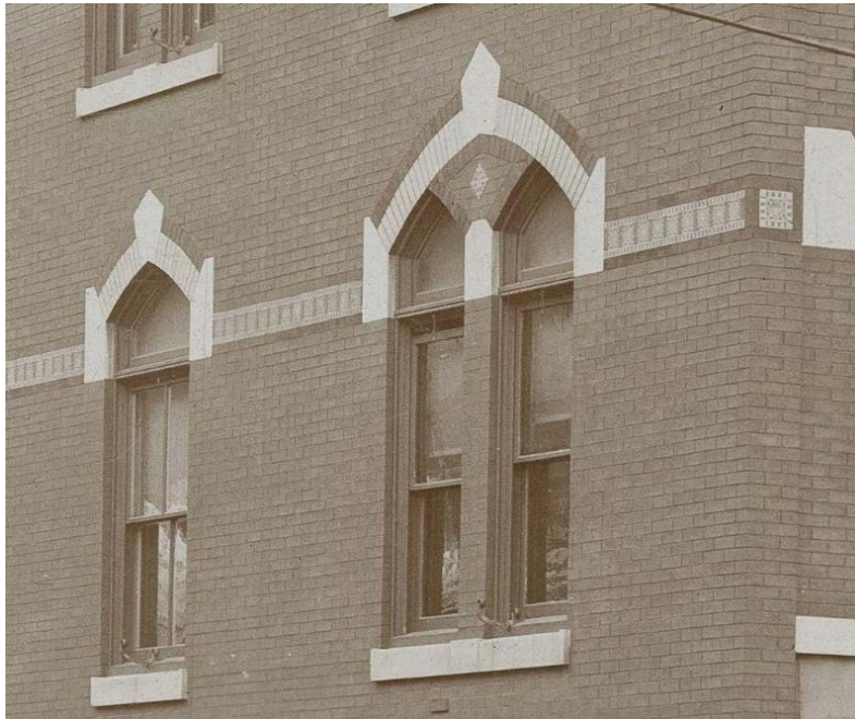
Figure 38: Detail of a turn-of-the-century photo shows the tile before it was painted over, as well as the window arrangement which previously existed on the right-most bay on the 11th Street elevation.
