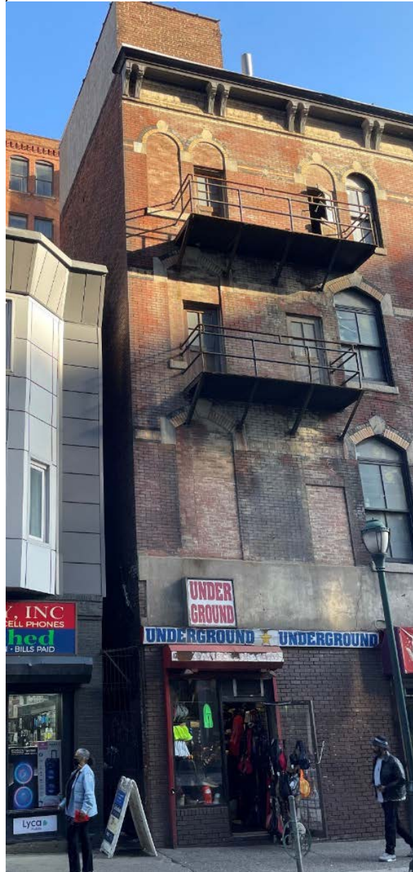
Figure 15: A narrow alley runs along the rear of 1039 Chestnut Street. The narrow aperture and debris in the alley make it difficult to photograph the North facade.
