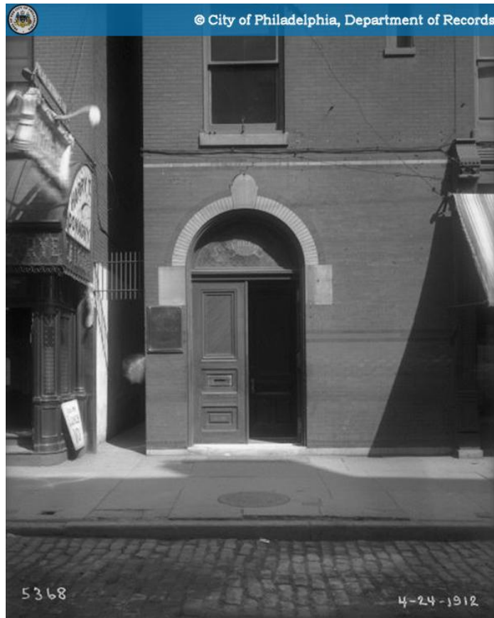
Figure 40: A photograph from 1912 shows decorative flourishes including polychrome banding.
