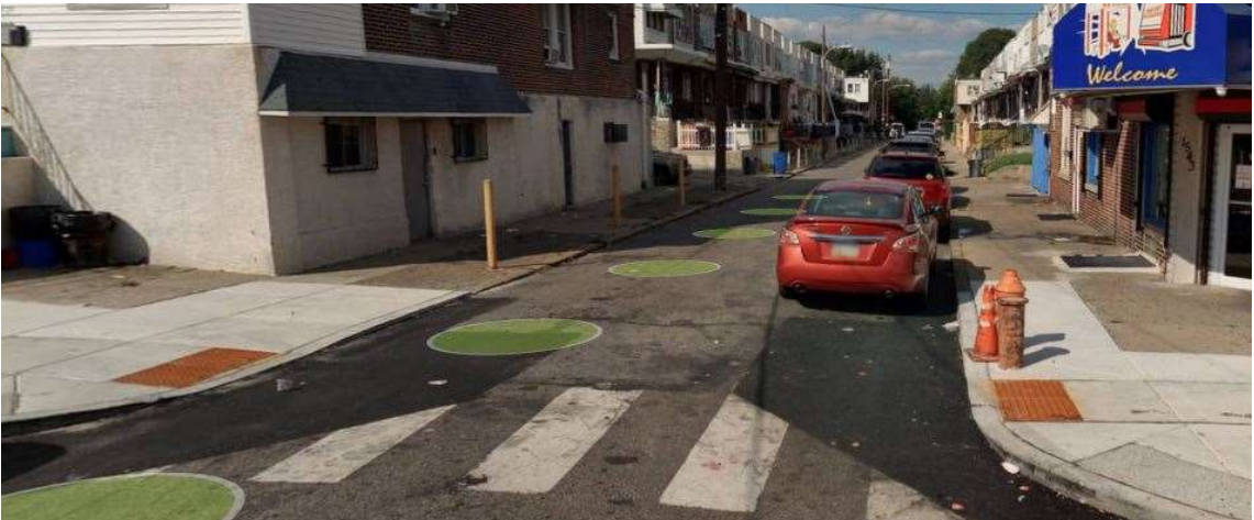
Before and After of Compliant ADA Curb at Luzerne St and Ormond Street
