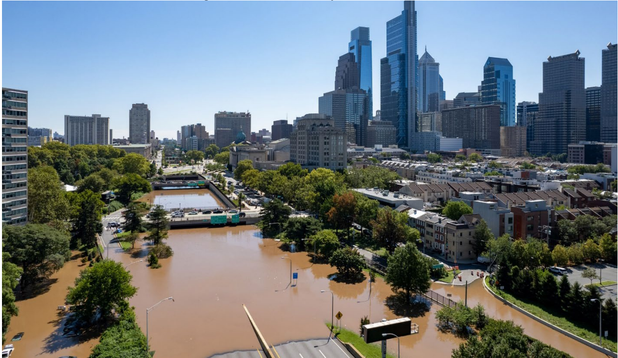
Figure 17: Interstate 676 after Hurricane Ida
