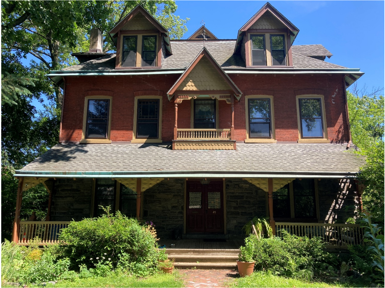
Figure 2: Front façade of 40 W Tulpehocken Street looking east, May 2024. Source: Author.
