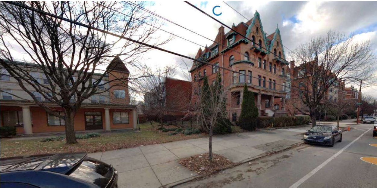
Figure 3: View of 4124-28 Parkside Ave looking Southwest from Parkside Ave.
