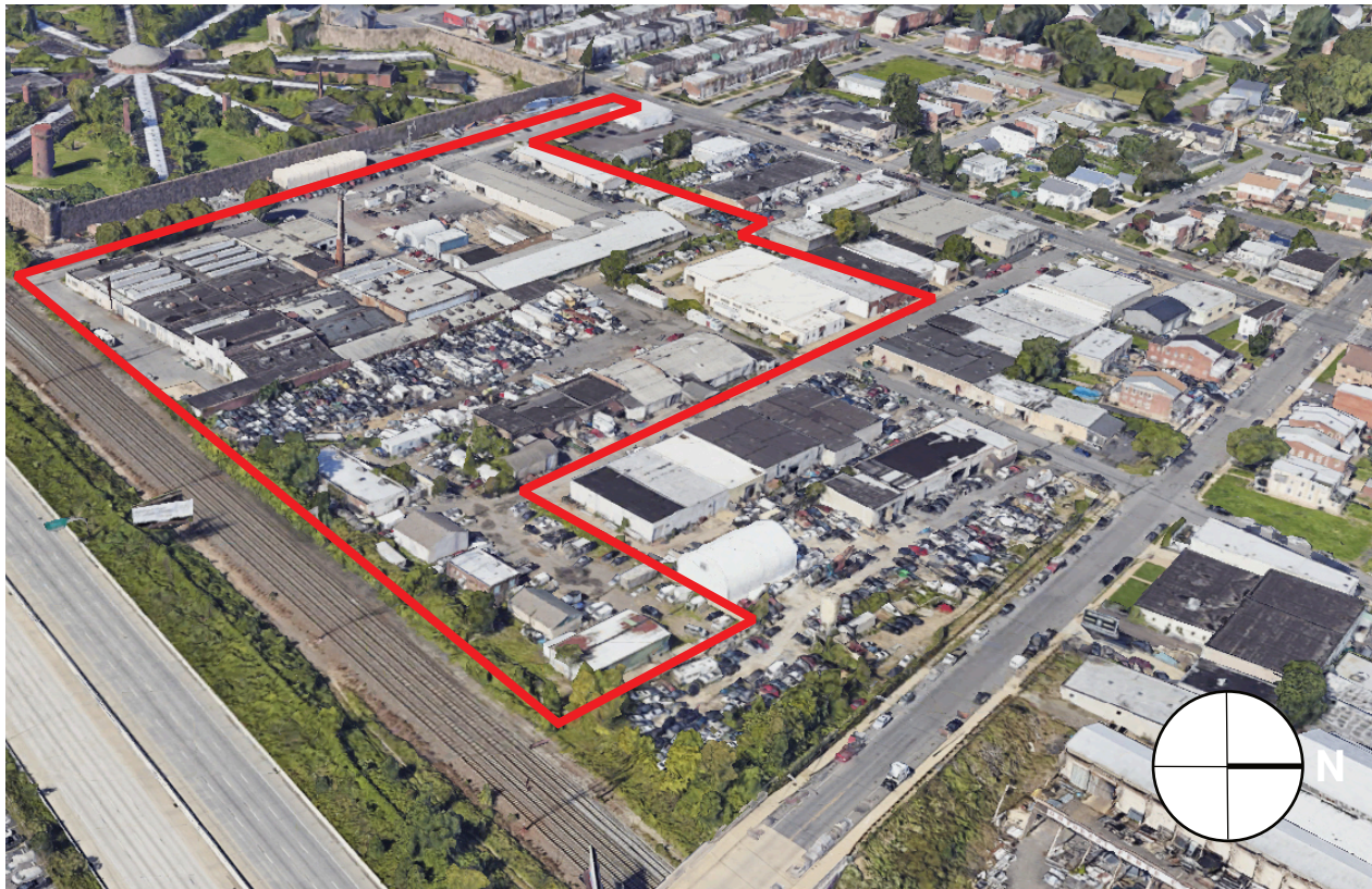
Aerial Photograph Looking West
