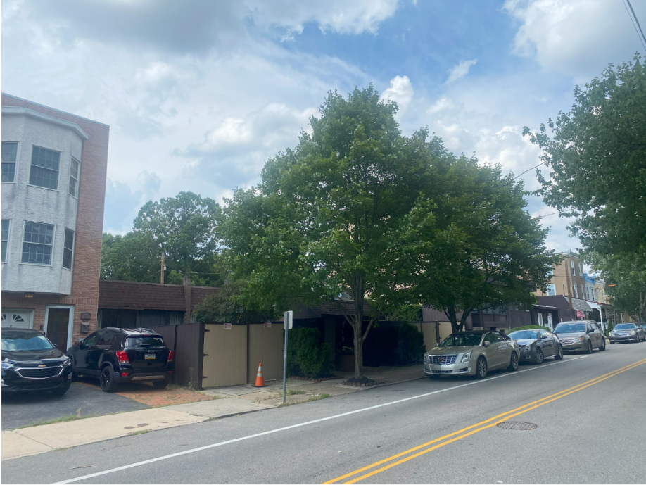
03 - MT PLEASANT AVE LOOKING WEST
