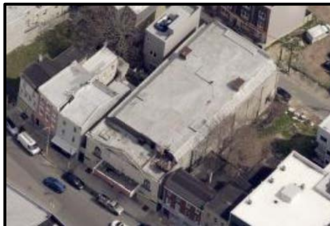
Figure 3. Looking east at the subject building. Source: Pictometry, Atlas, City of Philadelphia, 2024.
