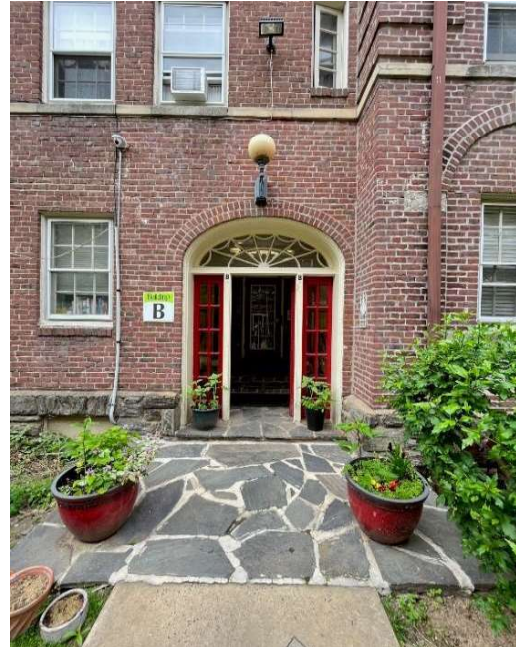
Typical Entry Detail View Image: Douglas Kingsbury
