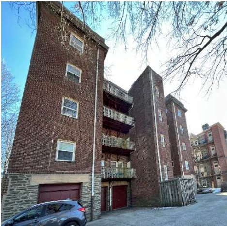
Rear Stair Towers: Libbie Hawes
