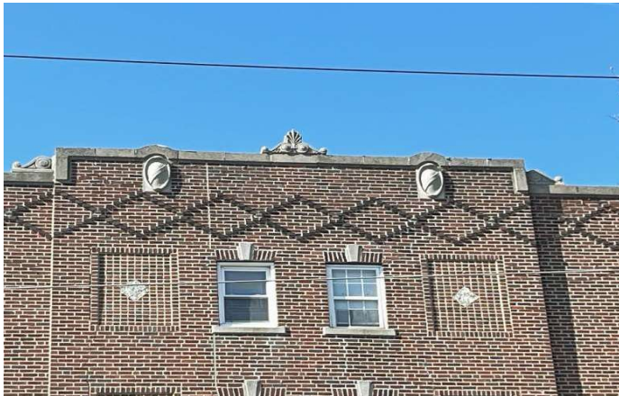
Rear Stair Towers: Libbie Hawes
