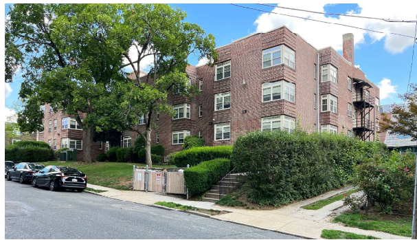
View of McCallum Street facade
