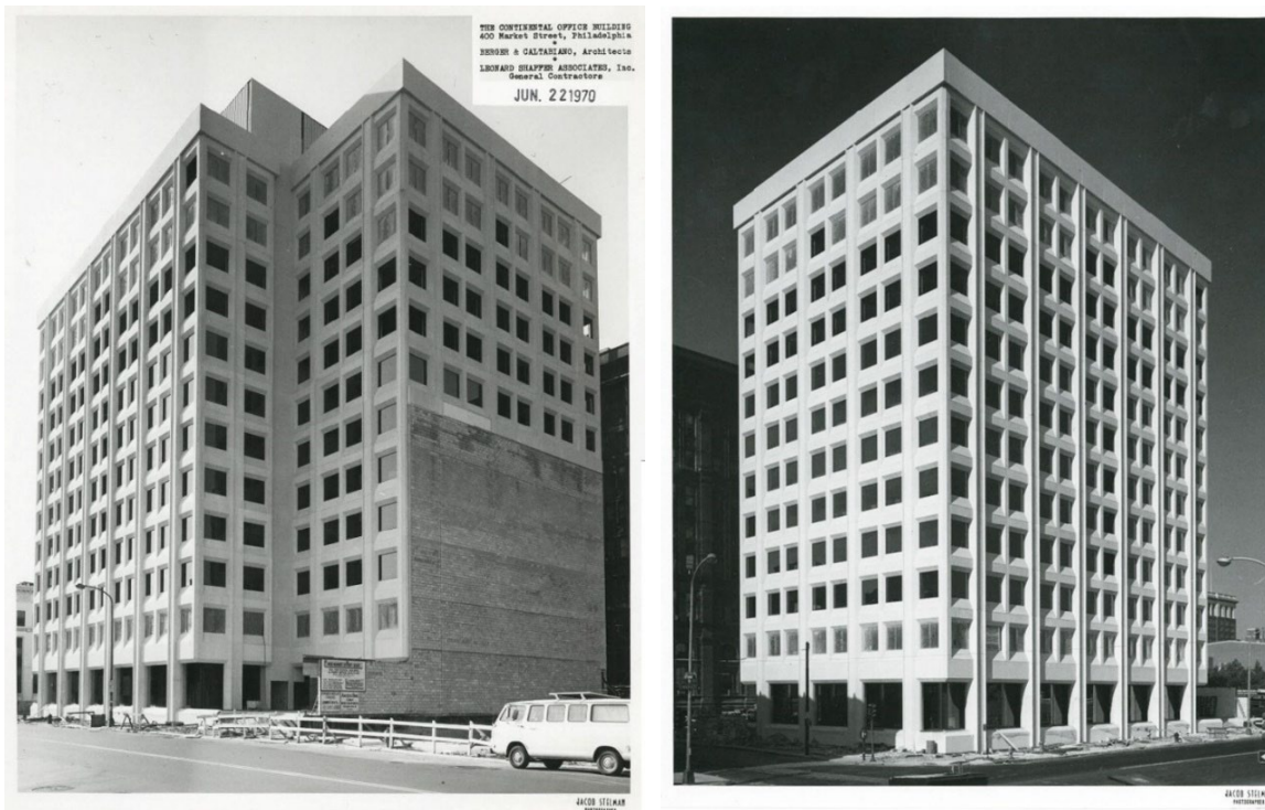
Figure 13: Two views of the Continental Building, looking southeast and southwest, respectively, in June 1970, shortly before it opened to tenants. Peter Olsen, photographer (from the Athenaeum of Philadelphia).
