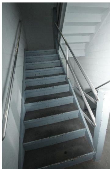
Photo 24 : 4th floor, fire stair at the southeast corner of the building.
