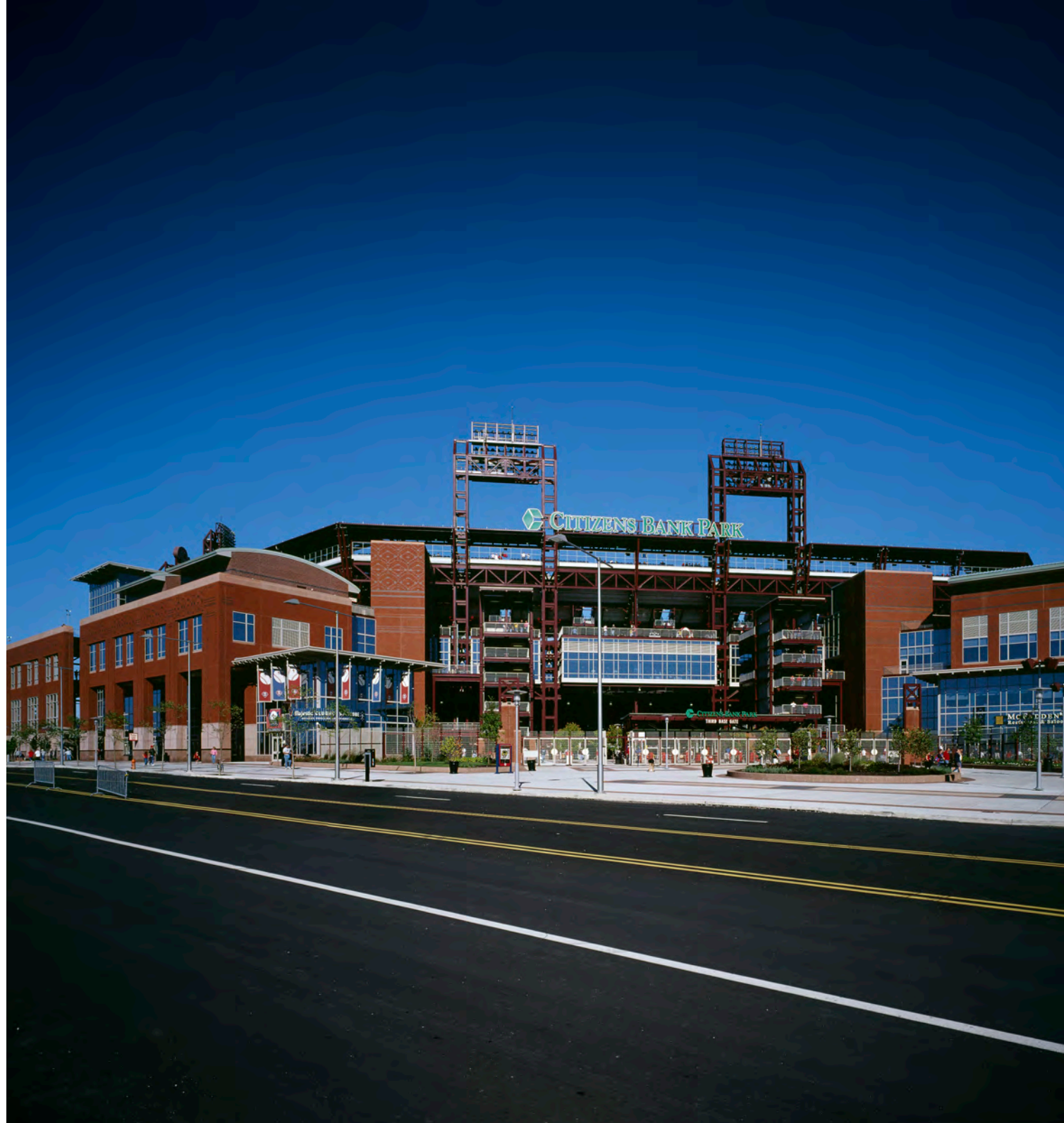
2004 view of 3rd base gate from CB Way
