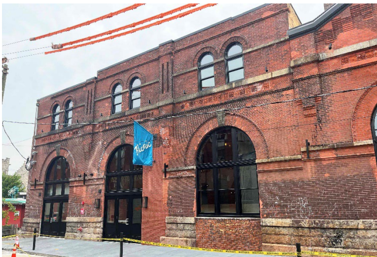
Photo 6: Storage Building, north elevation, looking south.
