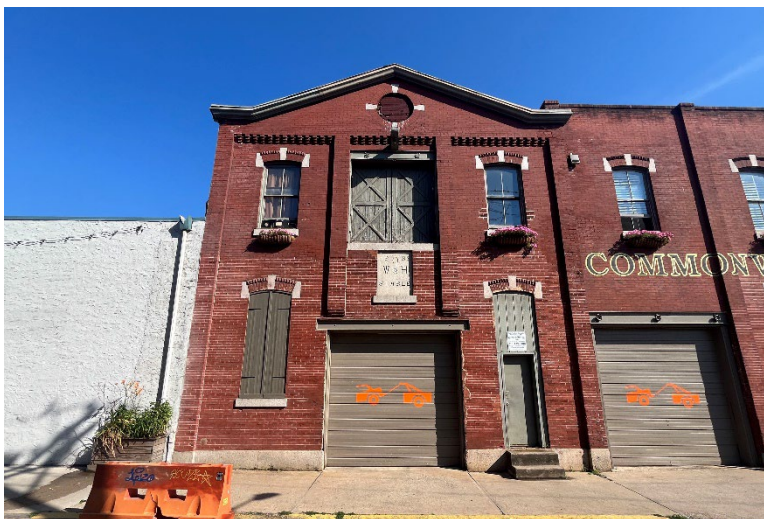
Photo 1: Stable A, south elevation of the original 1885 section, looking north.
