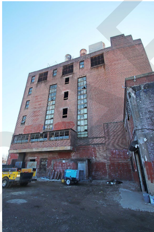
Photo 5: North elevation, looking south.
