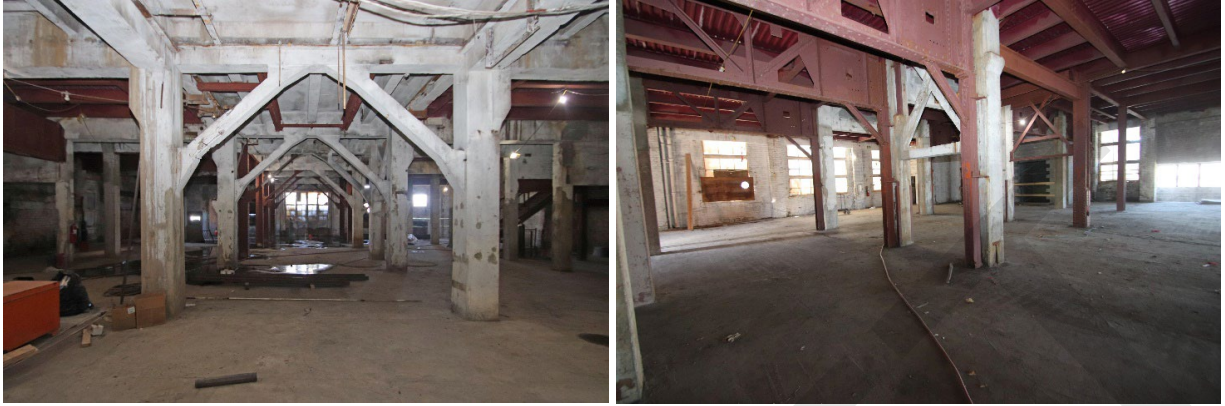
Photo 8: First floor, looking east. Photo 9: Second floor, looking northwest.
