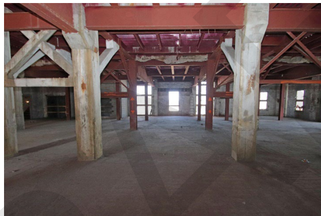
Photo 10: Fourth floor, looking north.
