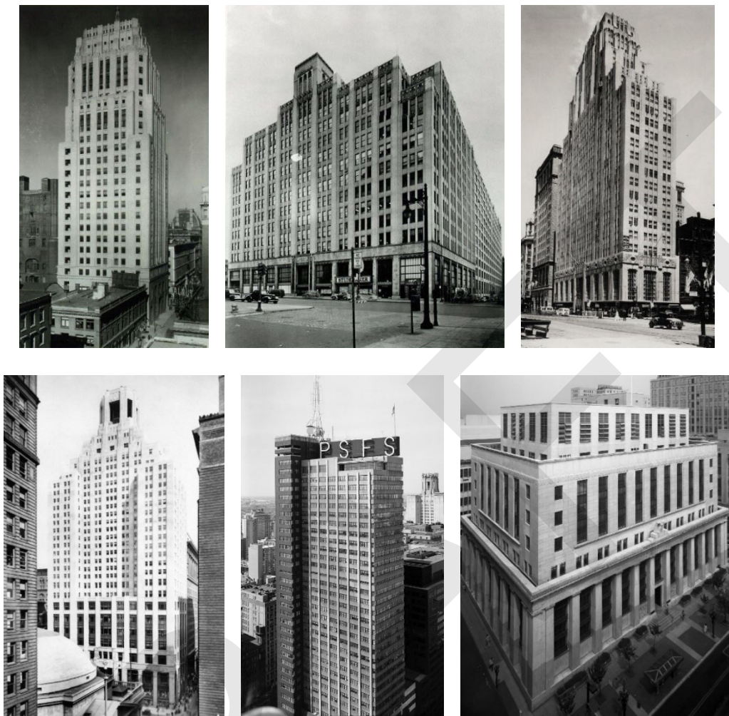
Figure 6: Six of the many large buildings that were heated with steam supplied by the Willow Steam Plant. From top left: The Philadelphia Electric Company Building, the Terminal Commerce Building, the Market Street National Bank, the Lincoln-Liberty Building, the PSFS Building, and the Federal Reserve Bank of Philadelphia (all images from the Athenaeum of Philadelphia except the PSFS Building, which is from the Library of Congress).
