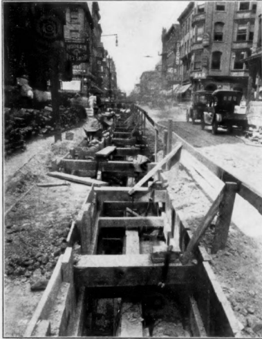
Figure 3: Construction of the steam main under 9th Street and details showing how the main was installed under the sidewalk (from Power Plant Engineering , October 15, 1927).
