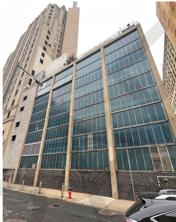
Figure 9: The Edison Steam Plant, built next to the headquarters of the Philadelphia Electric Company at 9th and Sansom Streets in 1958. Photo by the author.
