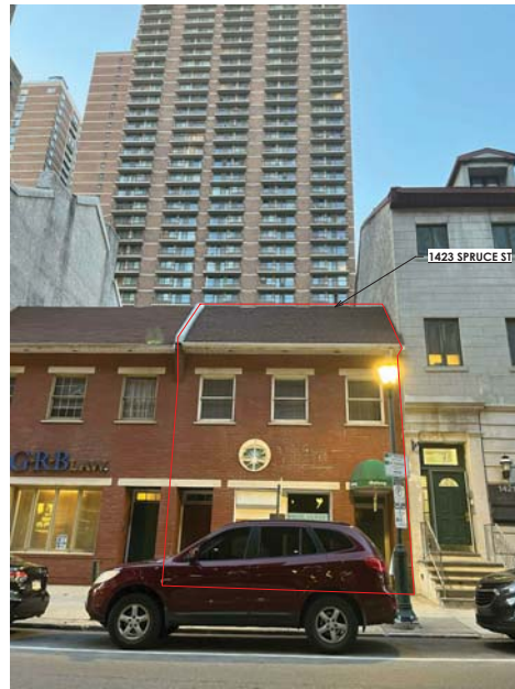
IMAGE 1: CURRENT CONDITION LOOKING NORTH AT SPRUCE ST
