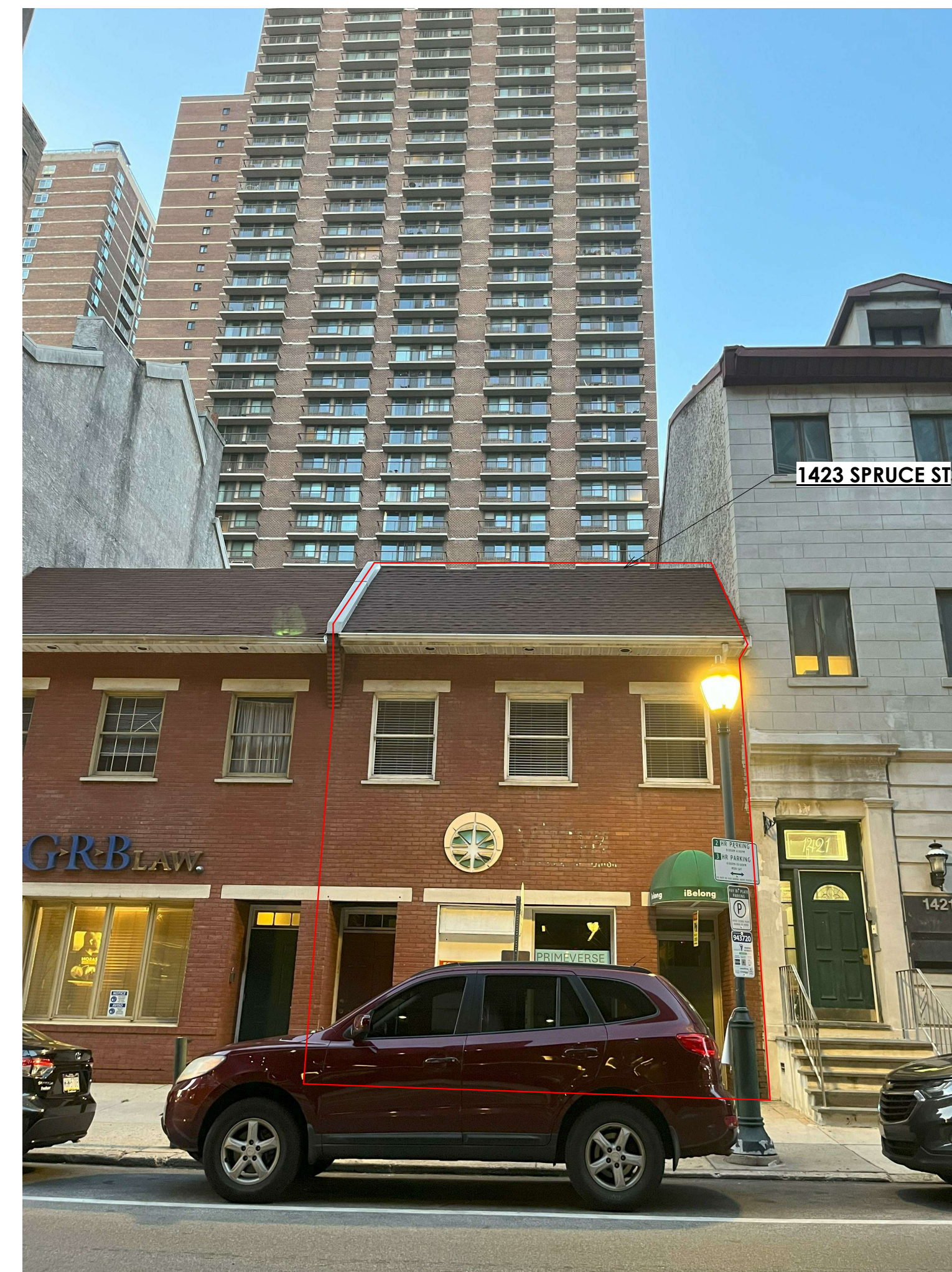
IMAGE 1: CURRENT CONDITION LOOKING NORTH AT SPRUCE ST
