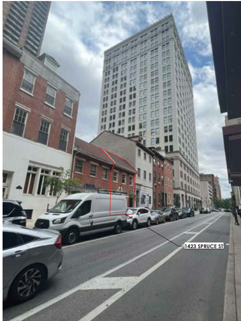
IMAGE 1: CURRENT CONDITION LOOKING EAST AT SPRUCE ST
