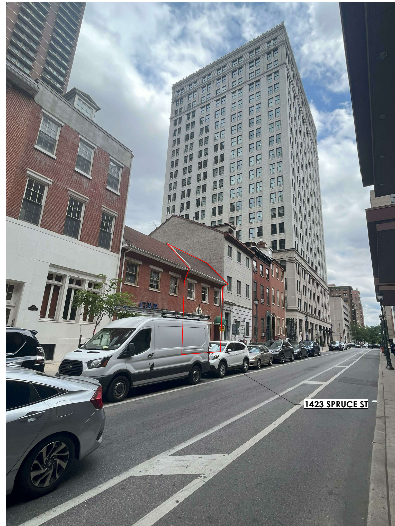
IMAGE 1: CURRENT CONDITION LOOKING EAST AT SPRUCE ST
