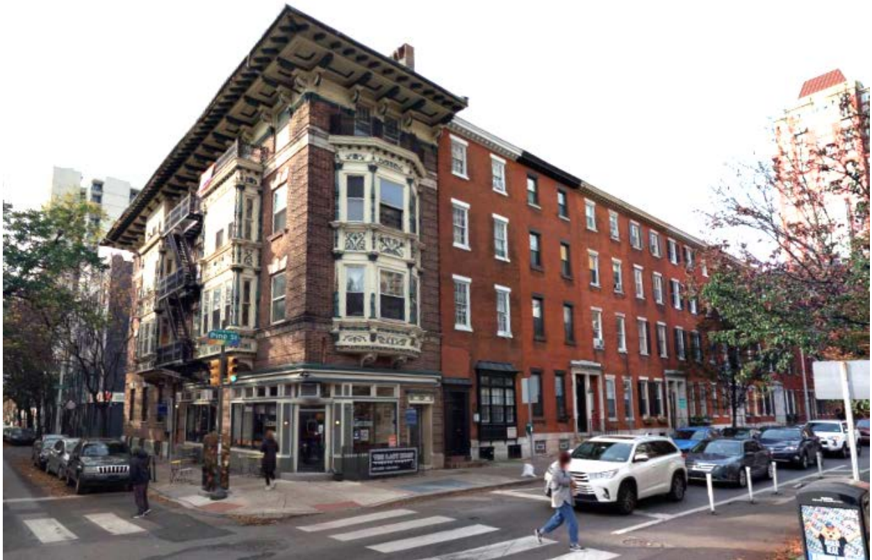
Photograph 14: Looking southwest along the 1300 block of Pine Street from S. 13 th Street. Cyclomedia, December 2021.
