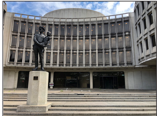
Plate 3: The original primary entrance on the north elevation. (Source: Allee Davis, June 2019)
