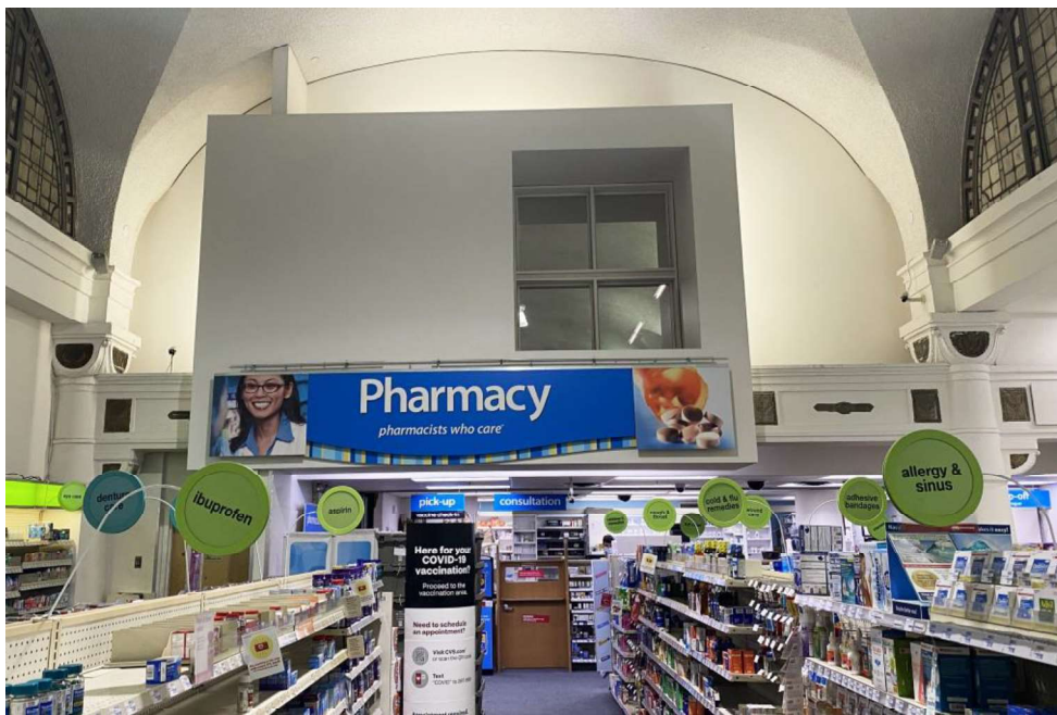
Figure 5a – South end of the Main Sales floor, looking south to the original mezzanine level, under which the pharmacy was located. The concrete frieze located behind the blue pharmacy sign is the lower edge of the mezzanine that was installed in 1913. The original inlaid Mercer tile details also remain, although the original iron mezzanine railing and the central stair leading up to the mezzanine were removed in recent decades.
