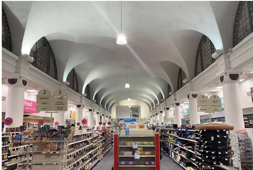
Figure 1 – Overall view of Main Sales Floor, looking south (October 2021). All photos were taken by the author, Kevin McMahon, unless otherwise noted. Refer to the plans in Figure 20 for photo locations.
