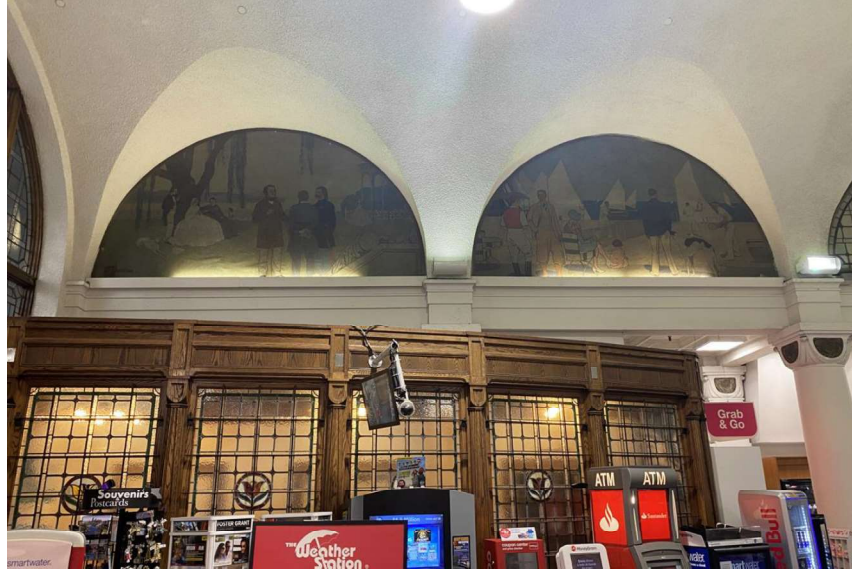
Figure 11 – View of east wall, columns 1-3 (left to right) showing the location of Murals 3 and 4.
