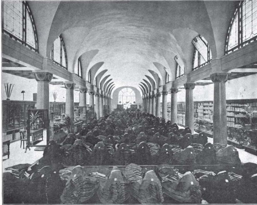
Figure 27 – Interior of the Main Sales Floor as pictured in the April 1905 edition of Men's Wear .
