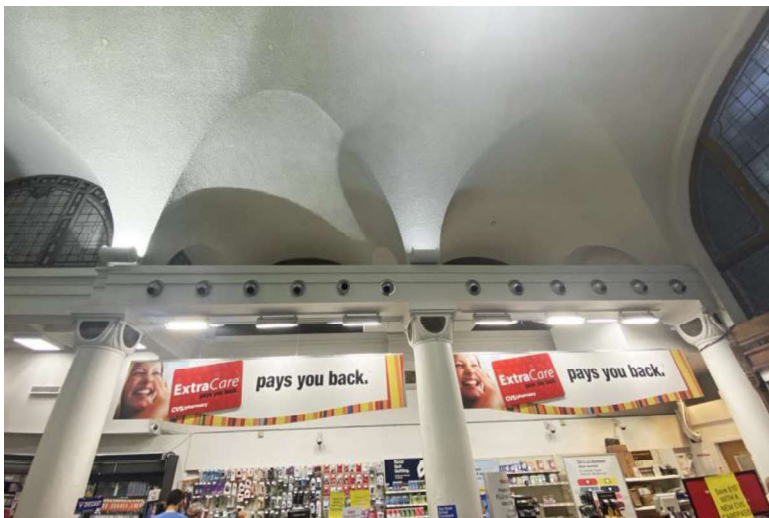
Figure 8 – View of west wall, columns 1-3 (right to left) showing the location of Murals 1 and 2.
