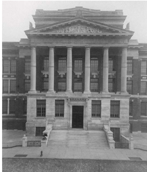
Figure 15 – Germantown High School, designed by Henry DeCoursey Richards and built in 1914-15, extant (Historic Germantown).
