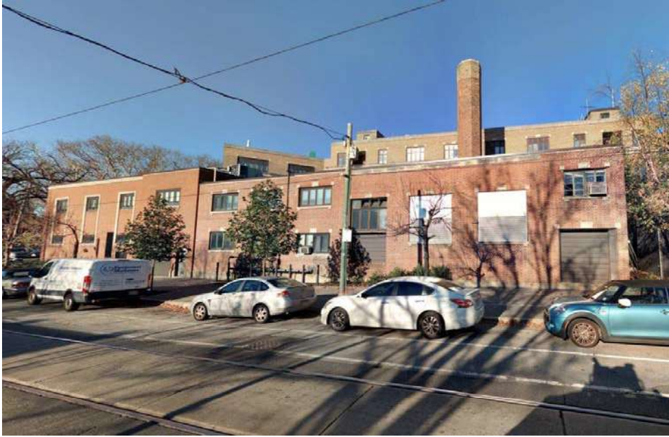
Figure 6 – South elevation of the 2-story boiler house addition, looking north from Woodland Avenue.
