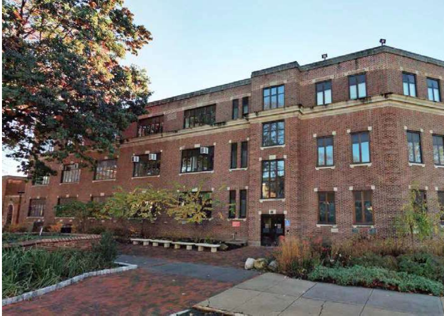
Figure 4 – North elevation, looking southeast from D'Angelo Mall (formerly Kingsessing Avenue).
