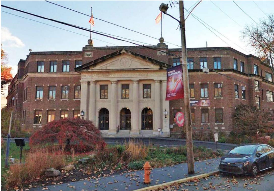
Figure 2 – Northwest elevation, looking southeast from 43rd Street.
