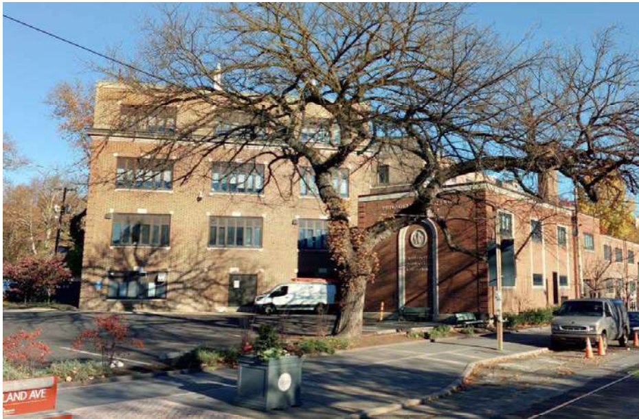
Figure 5 – South elevation of the 43rd Street wing, with the 2-story boiler house addition at right, looking north from Woodland Avenue.
