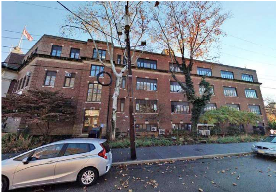
Figure 3 – West elevation, looking east from 43rd Street (formerly Kingsessing Avenue).
