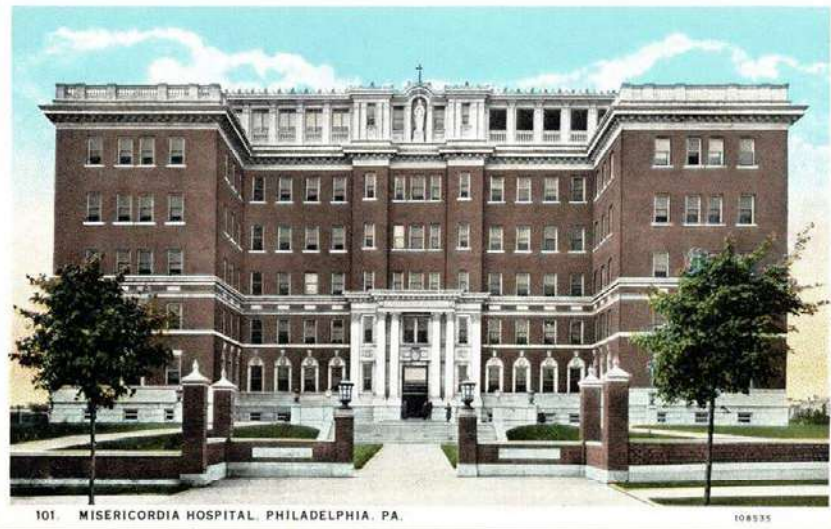
Figure 16 – Misericordia Hospital at 54th and Cedar Avenue, designed by F. Ferdinand Durang and built in 1915-24, extant.
