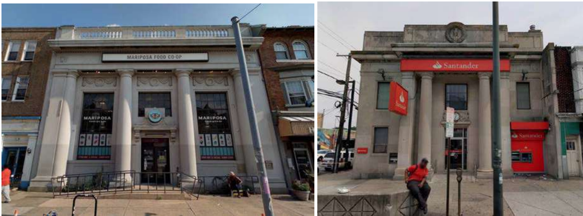
Figure 27 (left) – Belmont Trust Company (1923) at 4824 Baltimore Avenue in 2018 (Pictometry). Figure 28 (right) – Woodland Avenue State Bank (1925) at 65th and Woodland in 2018 (Pictometry).
