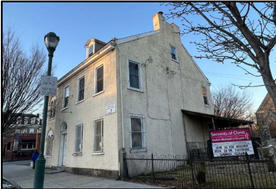
Figure 15. Top: The primary (southwest) elevation of the Fraley House, aka the Parsonage of St. Stephen's M. E. Church. Source: Oscar Beisert, 2023. Figure 16. Bottom: The primary (southwest) and side (southeast) elevations of the Fraley House, aka the Parsonage of St. Stephen's M. E. Church. Source: Oscar Beisert, 2023.
