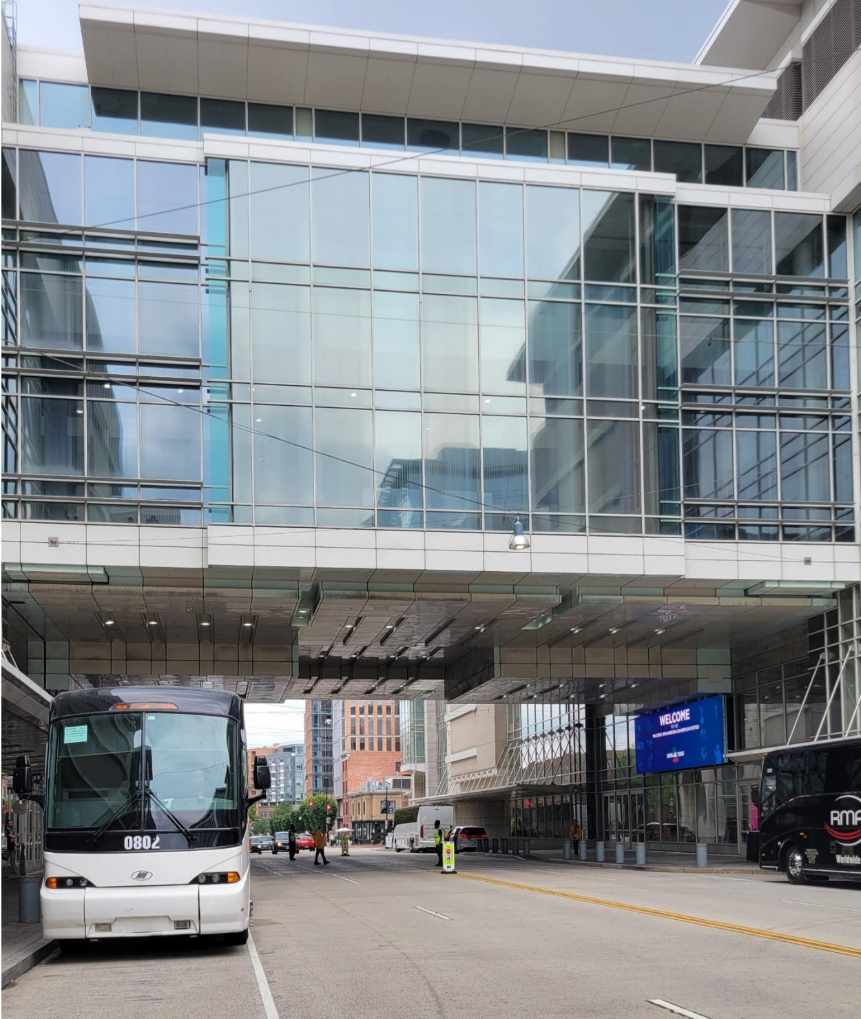
Building over street, Walter Washington Convention Center, Washington, D.C. Image source: Design Review Team
