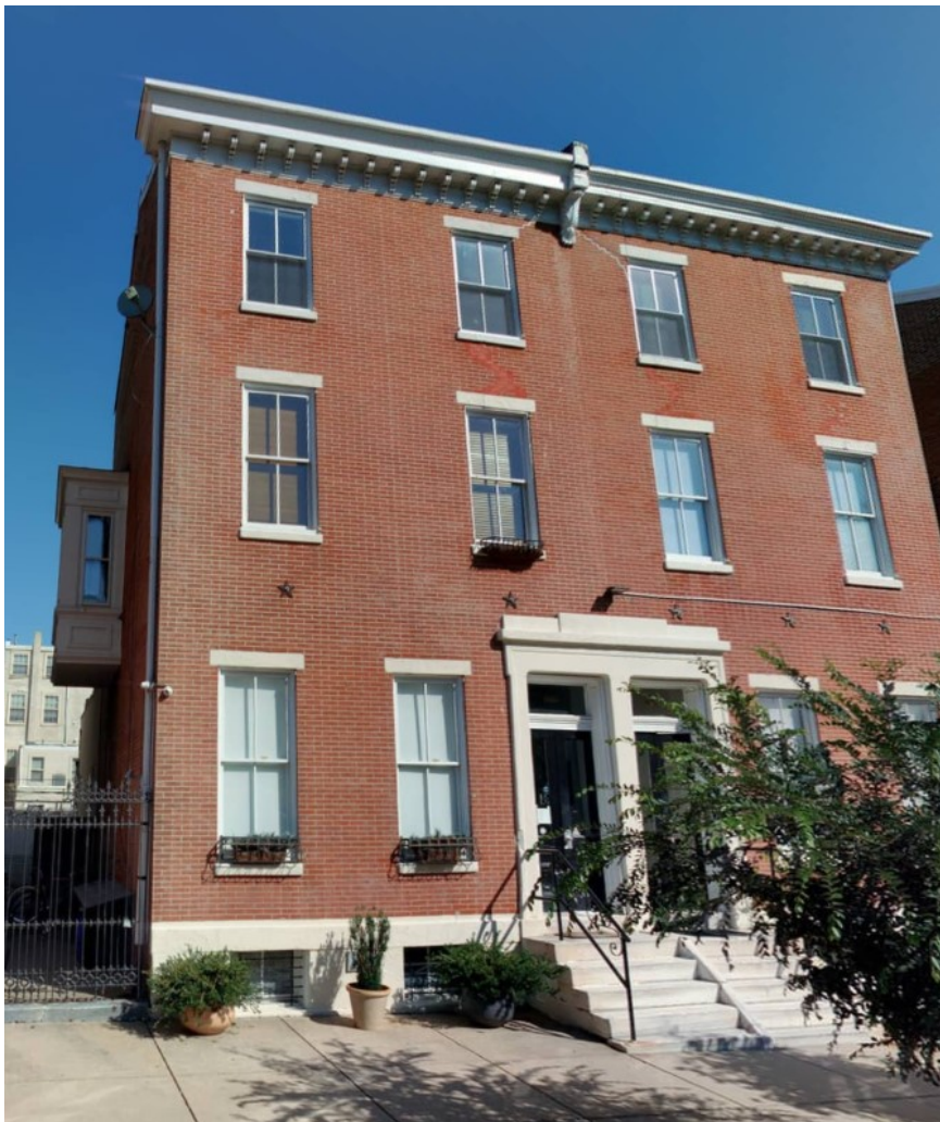
Figure 2: 1615 Green Street (left) primary elevation. The application proposes replacing the two 2 nd story windows. No work to side bay window.
