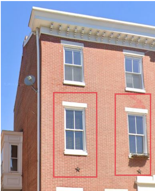
FRONT OF HOME CLOSE-UP VIEW OF 2 WINDOWS PROPOSED FOR REPLACEMENT
