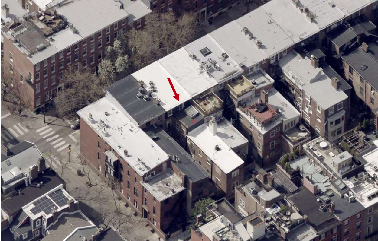
Figure 4: Aerial view of 1805 Pine St, looking southwest:
