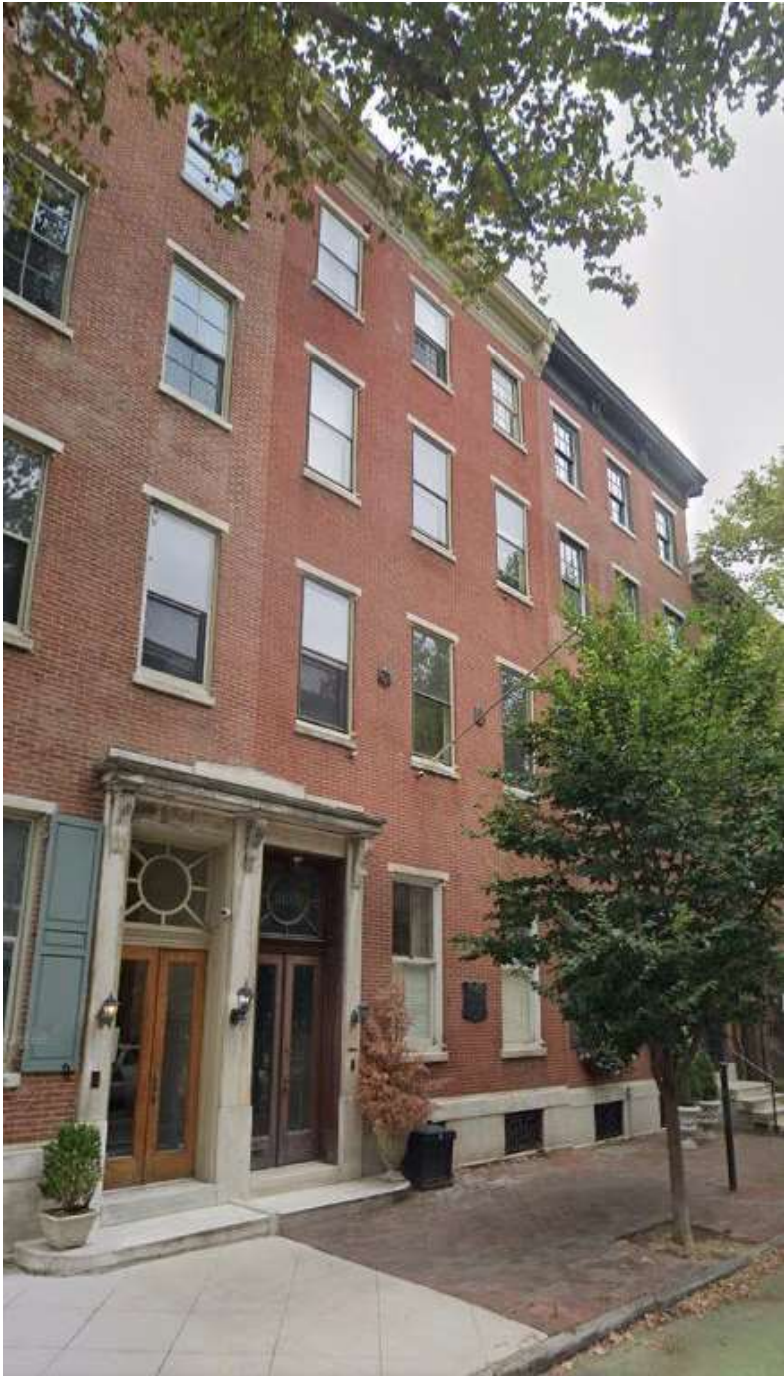
Figure 2: View of front façade of 1805 Pine St from Pine St:
