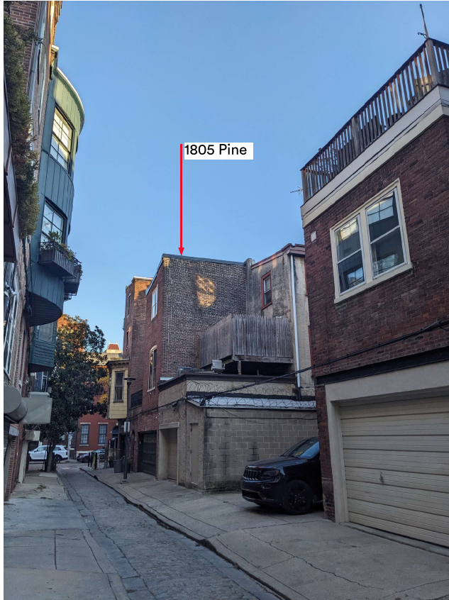
View from Panama St Existing
