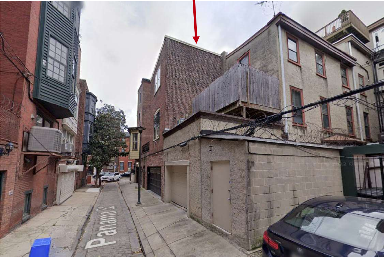
Figure 3: View looking west down Panama St, 1805 Pine indicated with red arrow:
