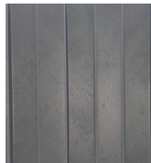
BOX RIB CORRUGATED METAL
