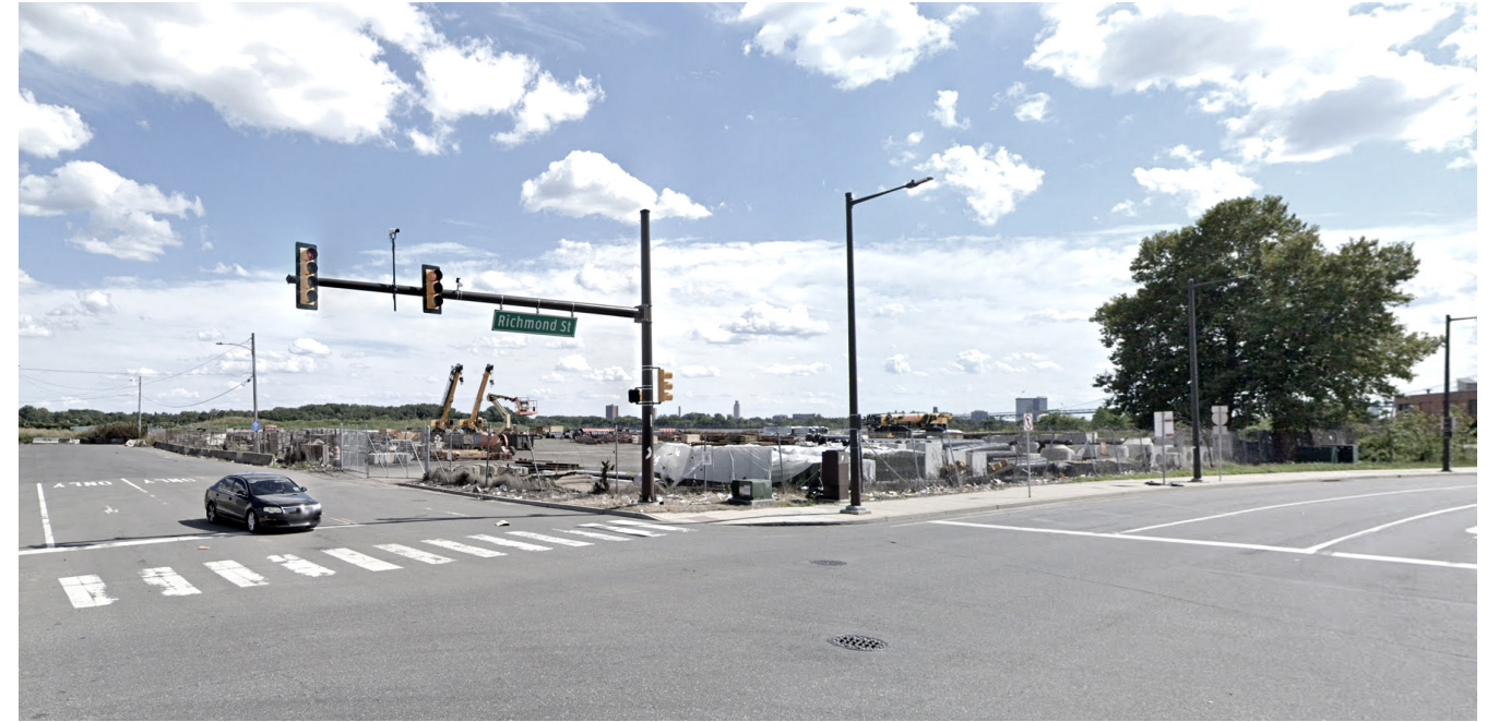
VIEW LOOKING S AT SCHIRRA + RICHMOND
