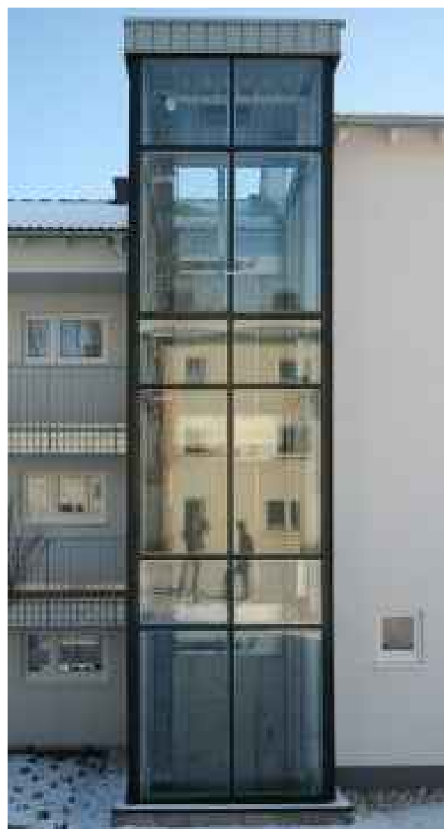
Glass Curtain Wall
