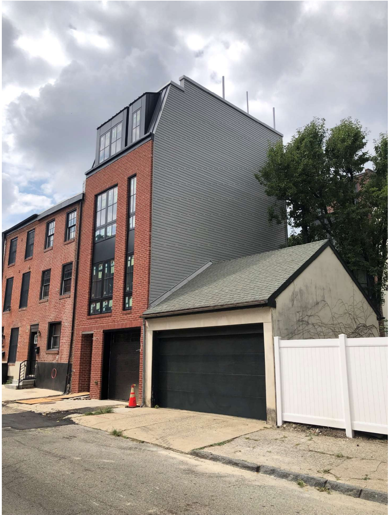
Figure 2. 1930 Pine Street rear along Waverly Street, July 2024.
