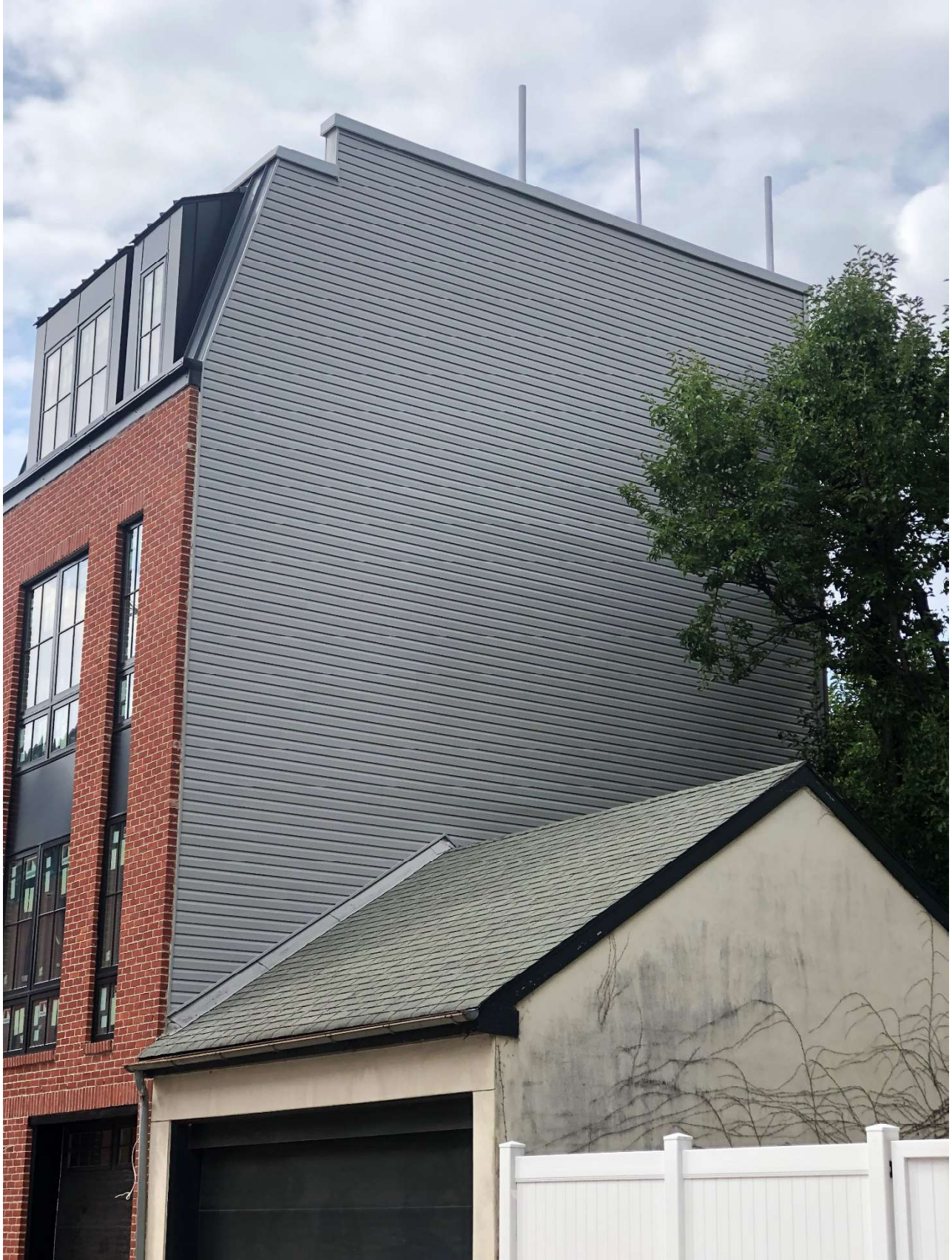
Figure 3. 1930 Pine Street rear along Waverly Street, showing side elevation of vinyl siding and lack of brick return. July 2024.
