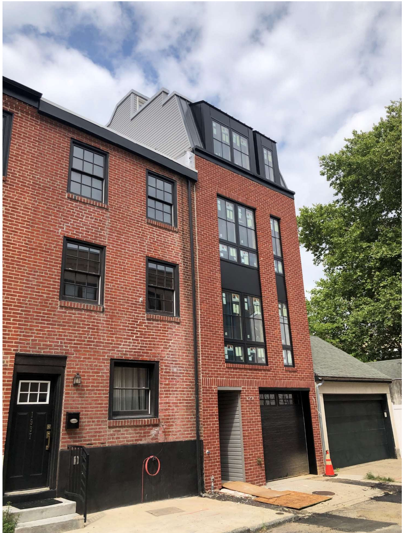
Figure 1. 1930 Pine Street rear along Waverly Street, July 2024.
