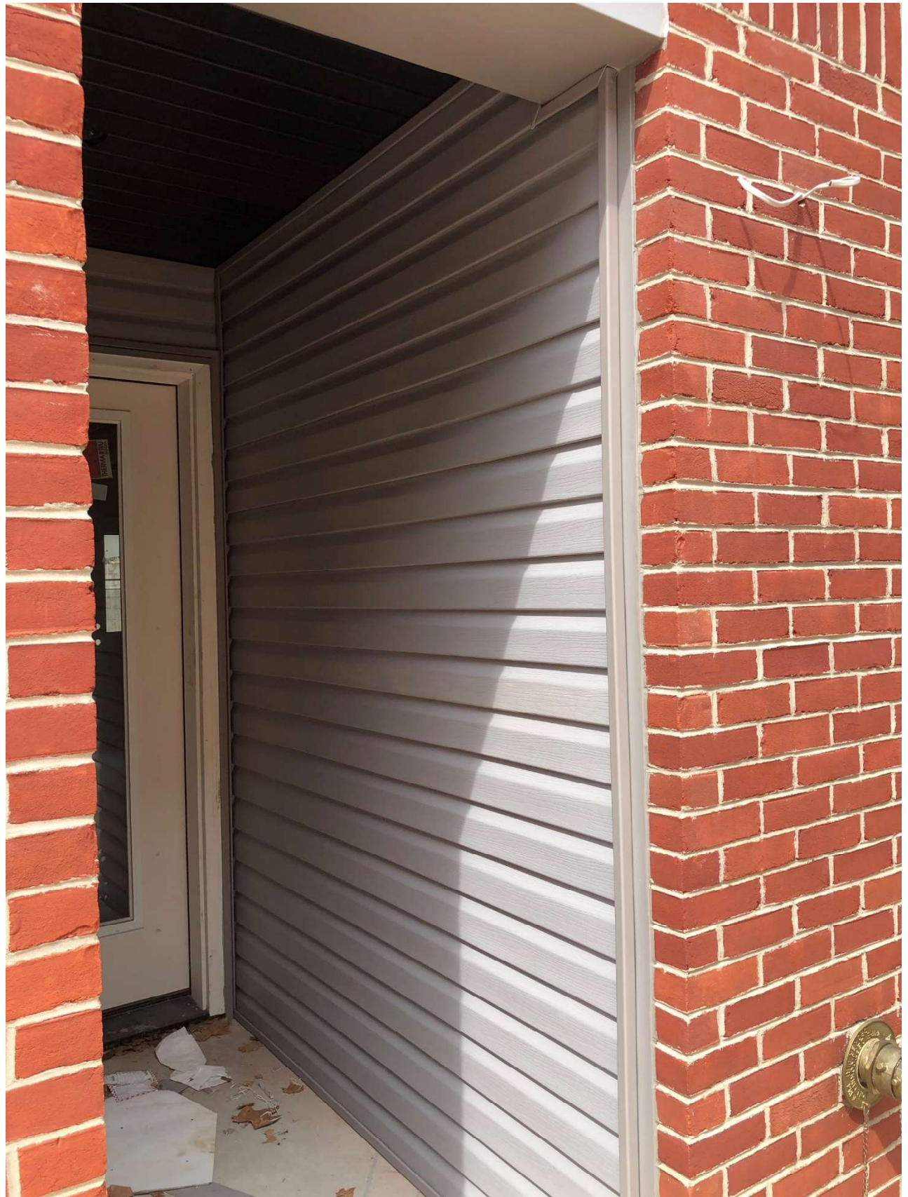
Figure 5. 1930 Pine Street rear along Waverly Street, showing vinyl siding at recessed entry. July 2024.
