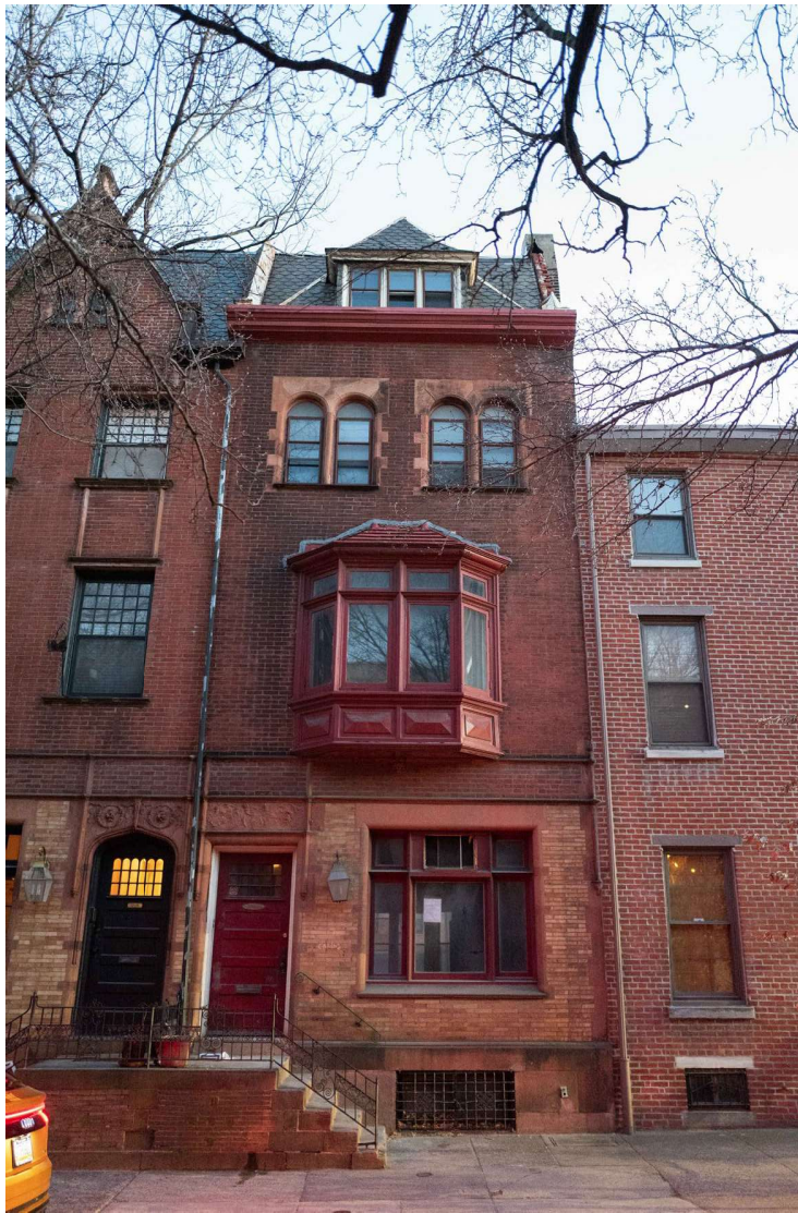
EXISTING FRONTAGE PINE ST (FOUR STORY MULTIFAMILY TO REMAIN)
