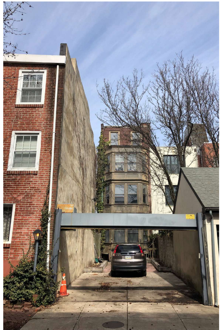
PREVIOUS FRONTAGE WAVERLY ST (SITE OF NEW CONSTRUCTION)
