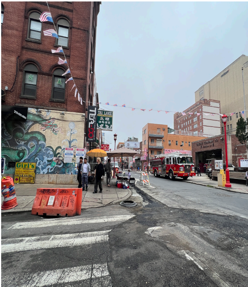
View of 10th and Cherry Street in Chinatown, facing north Source: BJH Advisors
