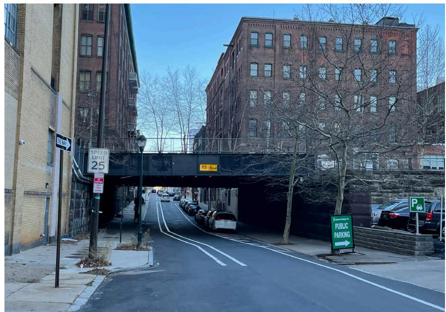
View of pedestrian underpass on 13th Street near Callowhill Street
