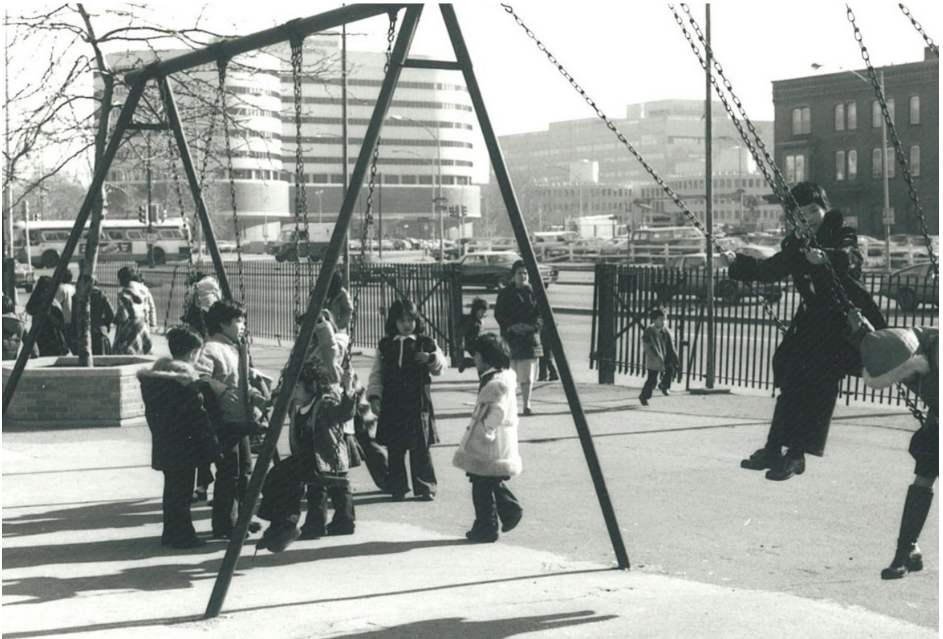
Holy Redeemer Church & School before the construction of the Vine Street Expressway Source: Philadelphia Chinatown Development Corporation
