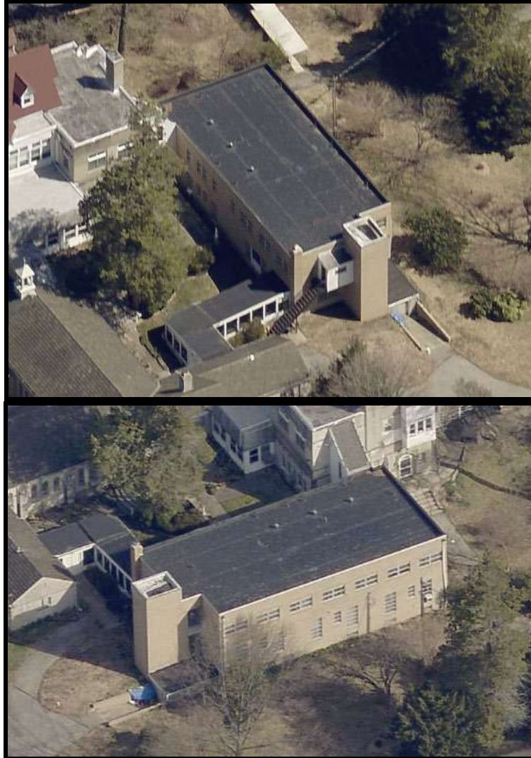
Figure 62. Top: The northwest and southwest elevations of the 1f. Dormitory. Figure 63. Bottom: The southwest and southeast elevations of the 1f. Dormitory. Source: Oscar Beisert, 2019.
