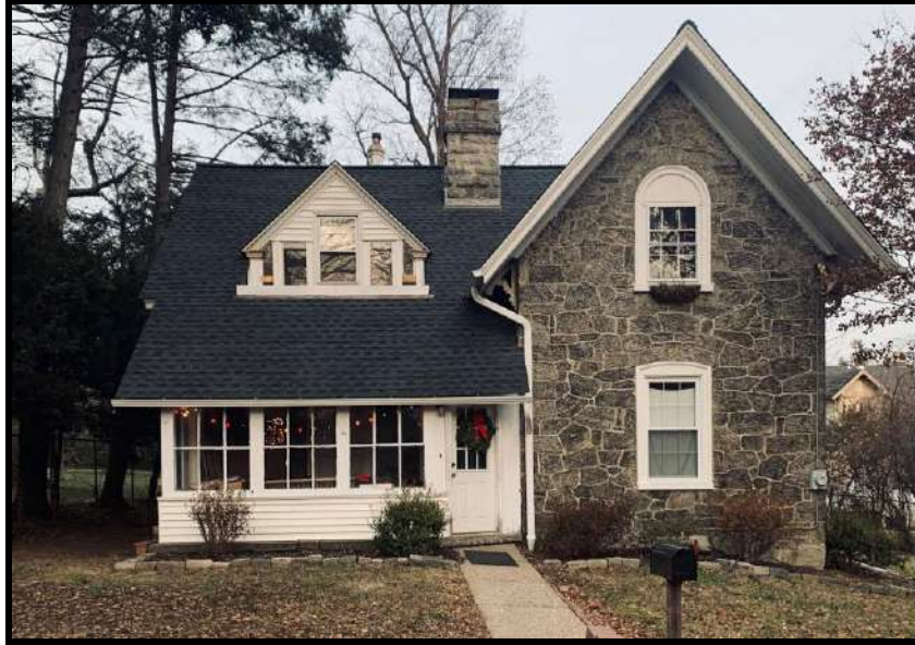
Figure 64. The primary (southwest) elevation of the Gardener's Cottage. Source: Oscar Beisert, 2019.
