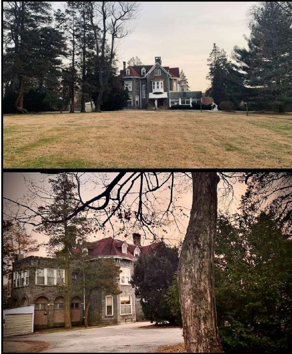
Figure 44. Top: The primary (northwest) elevation of the Main Block. Figure 45. Bottom: The northwest and northeast elevations of the Main Block from the driveway. Source: Oscar Beisert, 2019.
