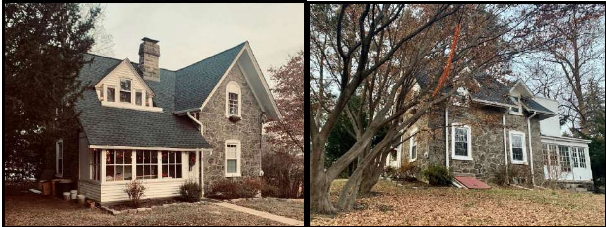
Figure 65. Left: The side (northwest) and primary (southwest) elevations of the Gardener's Cottage. Figure 66. Right: The primary (southwest) and side (southeast) elevations of the Gardener's Cottage. Source: Oscar Beisert, 2019.
