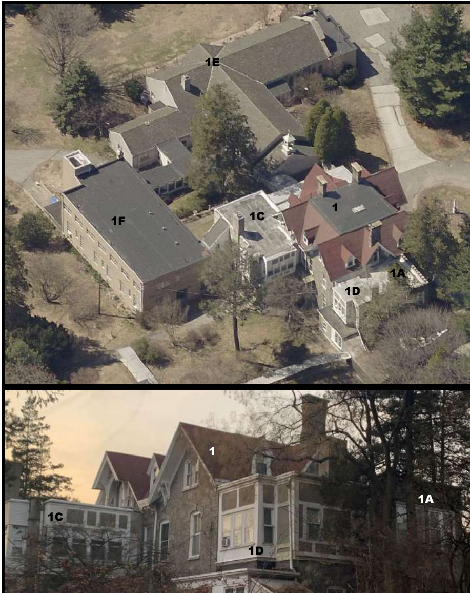
Figure 54. Top: Looking northwest at the Main Block and 1a. Arcade Addition, 1b. Porch Addition, 1c. East Addition, 1d. South Addition, 1e. Chapel Addition, and 1f. Dormitory. Source: Pictometry, Atlas, City of Philadelphia, 2019. Figure 55. Bottom: The rear (southeast) and side (northeast) elevations of the Main Block with 1c. East Addition, 1d. South Addition, and 1a. Arcade Addition also in view. Source: Oscar Beisert, 2019.
