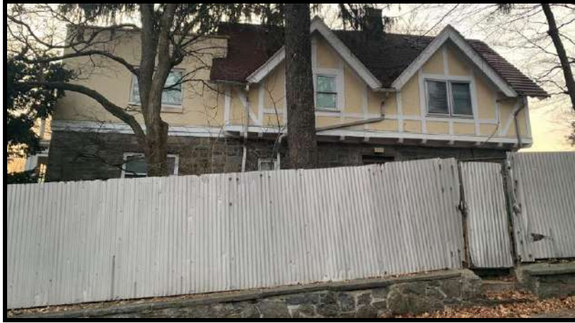
Figure 74. The primary (northeast) elevation of Cherry Cottage. Source: Oscar Beisert, 2019.
