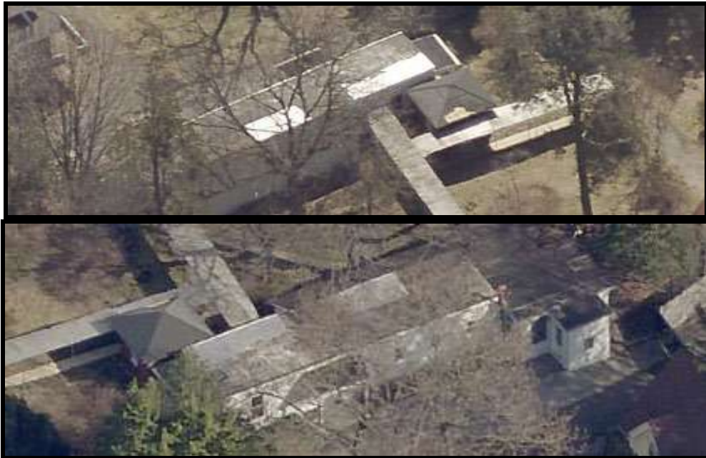
Figure 77. Top: The northwest elevation of the Garden Buildings A & B. Figure 78. Bottom: The rear elevation of the Garden Buildings A & B. Source: Pictometry, Atlas, City of Philadelphia, 2019.
