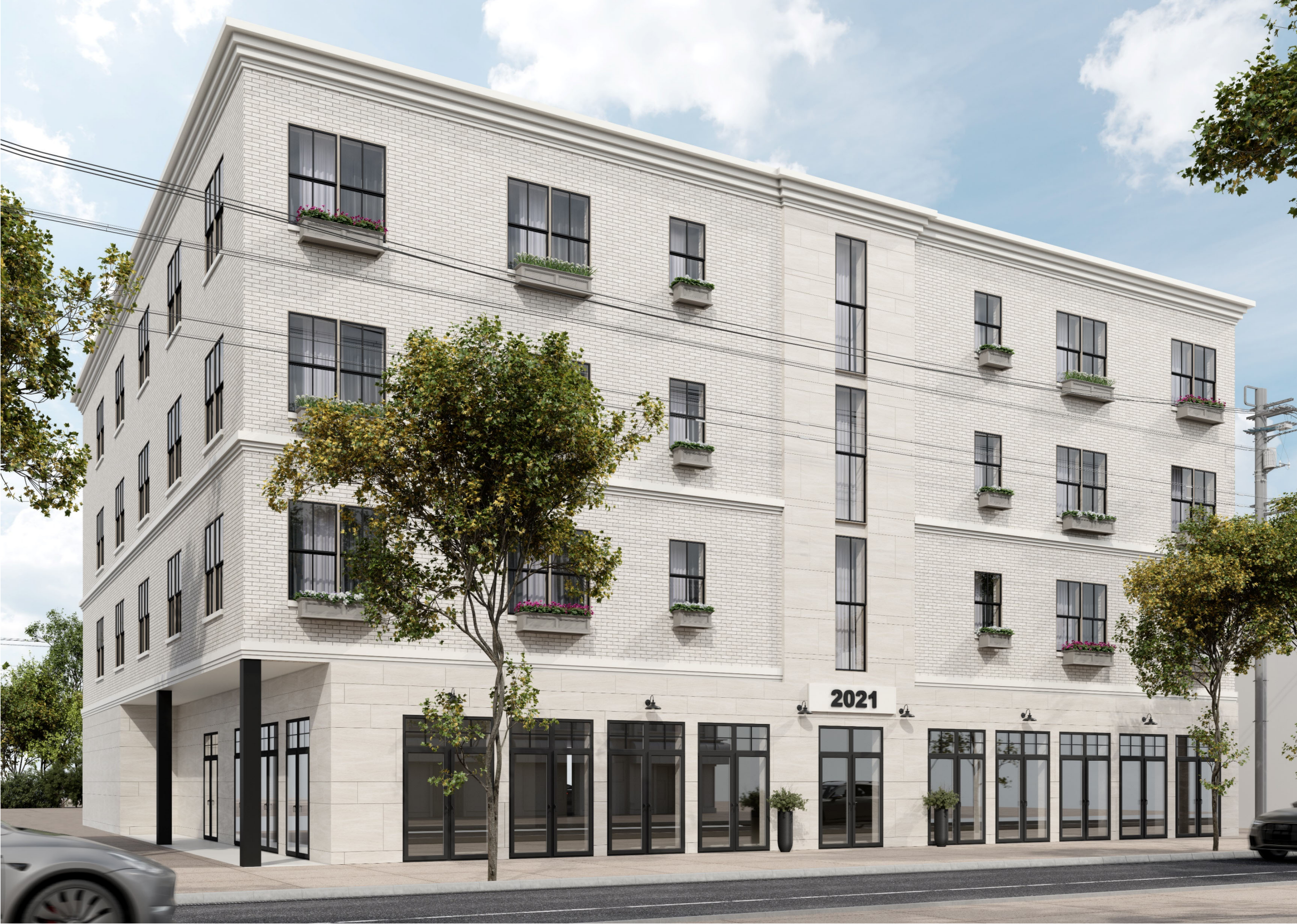
View of complex from N 63 rd Street
