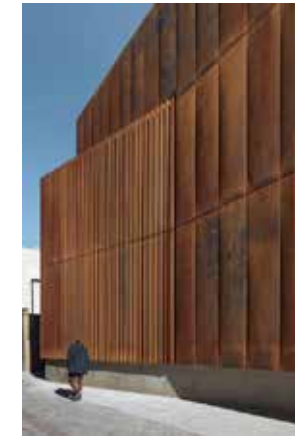
4 WEATHERED STEEL PANEL WEATHERED CORTEN STEEL PANELS WITH SMOOTH FINISH AND EXPOSED FASTENERS
