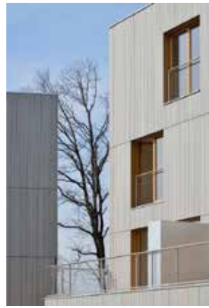
3 CORRUGATED METAL PANEL LIGHT GRAY ALUMINUM COMPOSITE PANEL WITH CORRUGATED FINISH, VERTICAL APPLICATION
