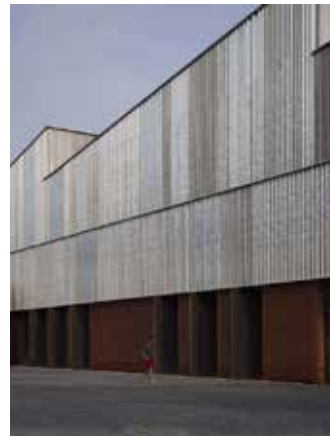
3 CORRUGATED METAL PANEL LIGHT GRAY ALUMINUM COMPOSITE PANEL WITH CORRUGATED FINISH, VERTICAL APPLICATION
