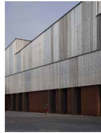
3 LIGHT CORRUGATED METAL PANEL LIGHT GRAY ALUMINUM COMPOSITE PANEL WITH CORRUGATED FINISH, VERTICAL APPLICATION
