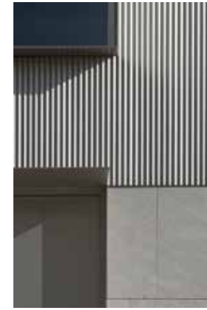
3 LIGHT CORRUGATED METAL PANEL LIGHT GRAY ALUMINUM COMPOSITE PANEL WITH CORRUGATED FINISH, VERTICAL APPLICATION
