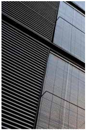
5 DARK CORRUGATED METAL PANEL CHARCOAL GRAY ALUMINUM COMPOSITE PANEL WITH CORRUGATED FINISH, VERTICAL APPLICATION
