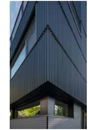
5 DARK CORRUGATED METAL PANEL CHARCOAL GRAY ALUMINUM COMPOSITE PANEL WITH CORRUGATED FINISH, VERTICAL APPLICATION
