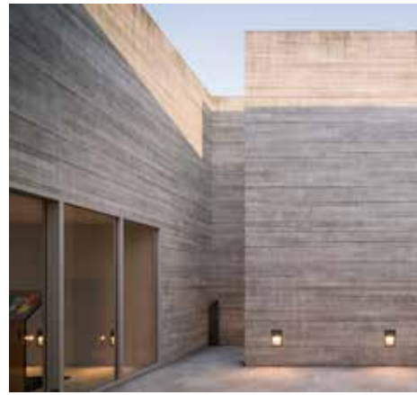
1 ARCHITECTURAL CONCRETE PRE-CAST CONCRETE WALL PANELS WITH NATURAL FINISH
