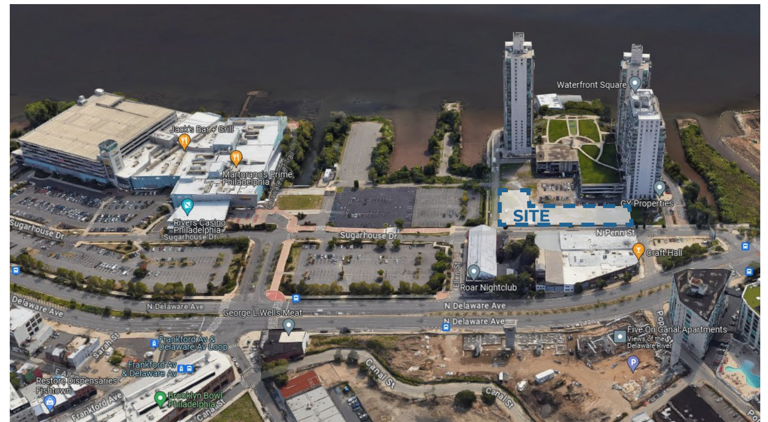
Looking East Of The Site
