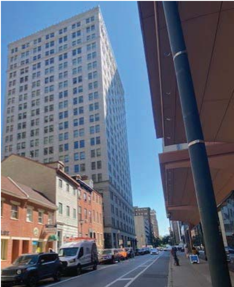
Figure 3. Spruce Street east of proposed building.
