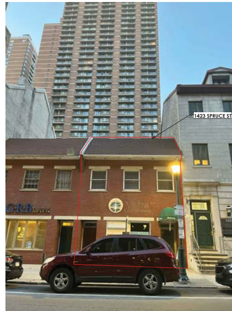
IMAGE 1: CURRENT CONDITION LOOKING NORTH AT SPRUCE ST
