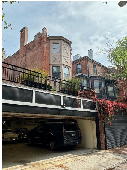
PHOTO: CYPRESS ST - LOOKING EAST
