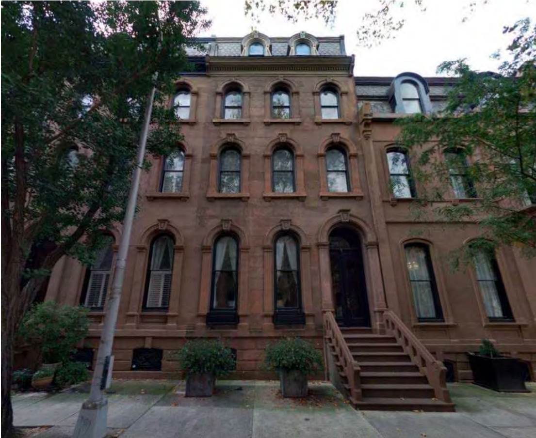
Figure 2: View of front façade of 2012 Spruce St from Spruce St:
