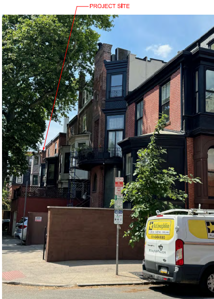
PHOTO: CYPRESS ST/20TH ST INTERSECTION
