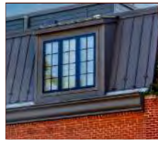
2. METAL STANDING SEAM MANSARD FOOR
