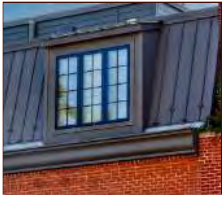
2. METAL STANDING SEAM MANSARD FOOR
