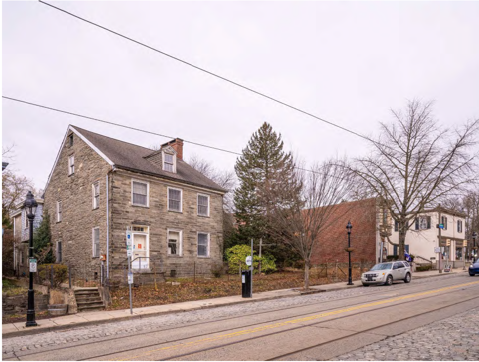
SITE PHOTO 1: LOOKING AT SOUTH-EAST SIDE OF THE SITE
