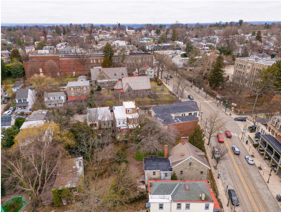
SITE PHOTO 1: LOOKING AT SOUTH SIDE OF THE BUILDING
