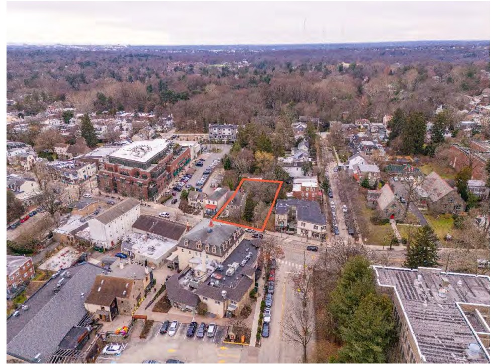
EXISTING AERIAL 2 : EAST
