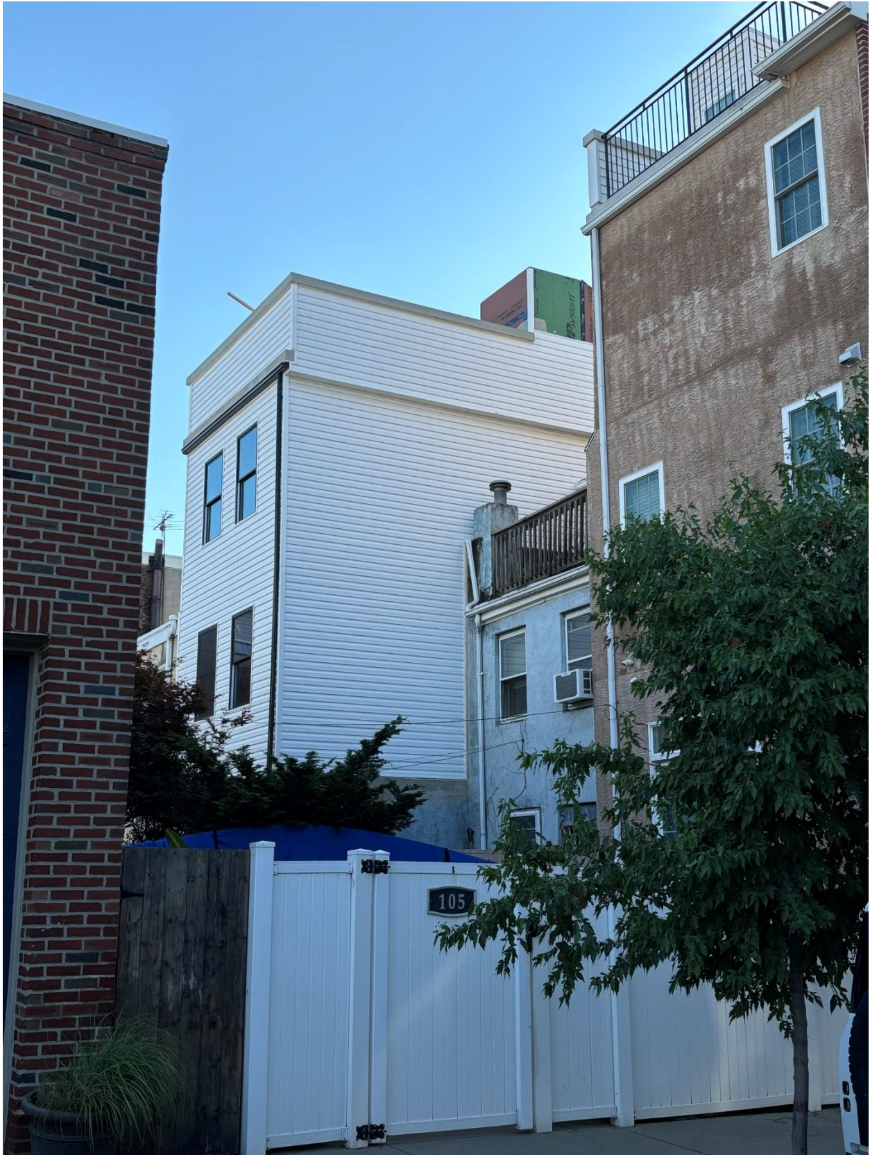
Rear of 1108 S. Front Street, 7/11/2024.
