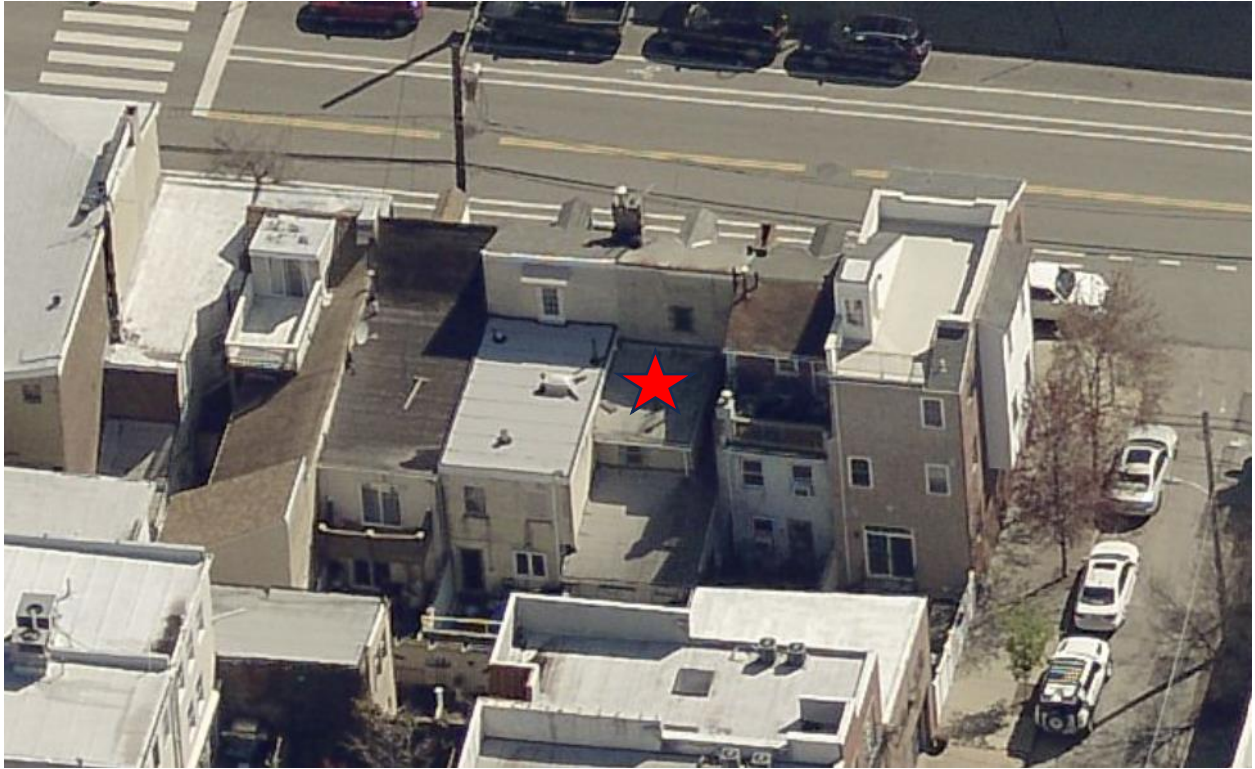
Aerial view of 1108 S. Front Street prior to recent work.
