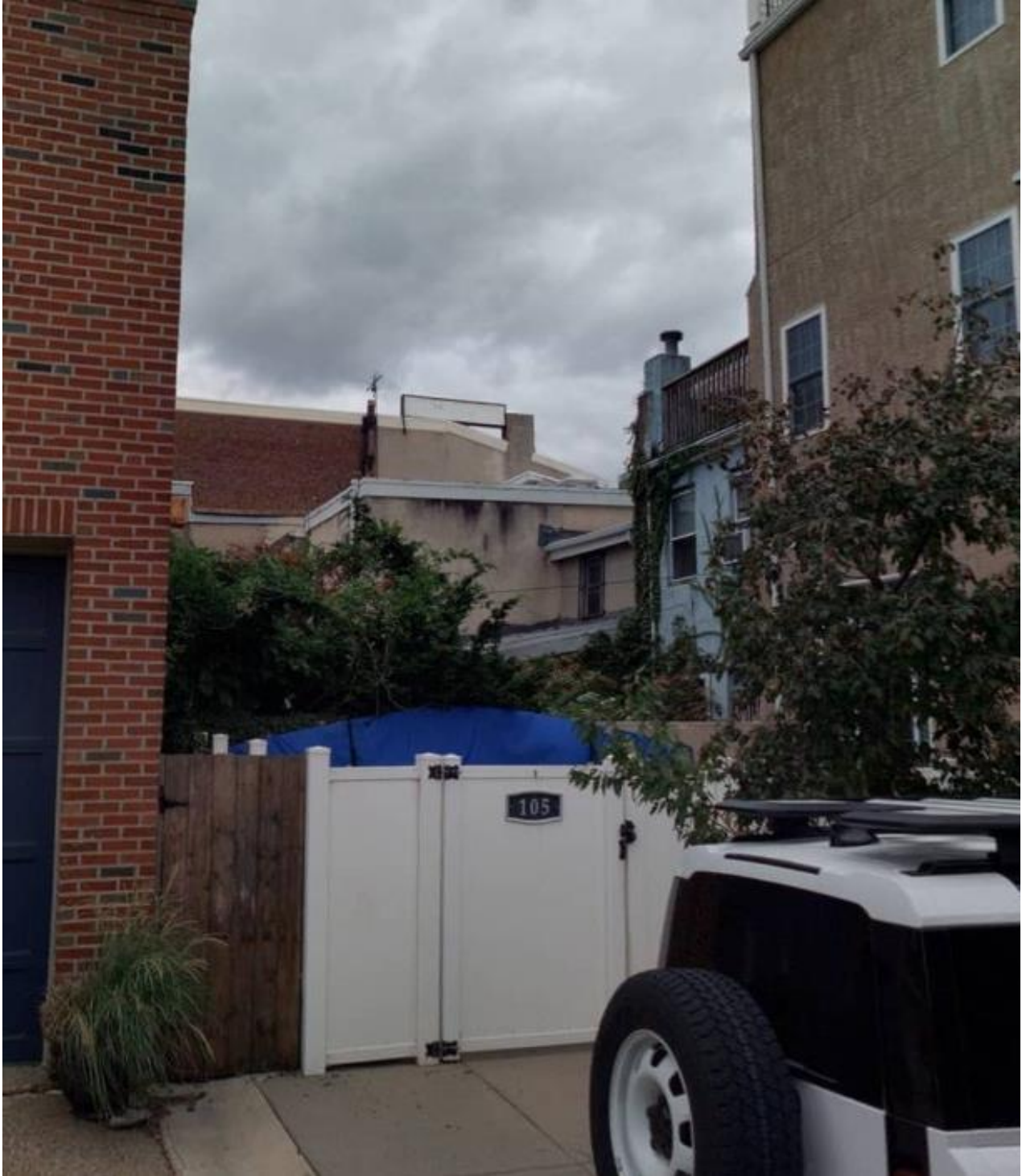
Rear of 1108 S. Front Street, 10/9/2023 prior to work.
