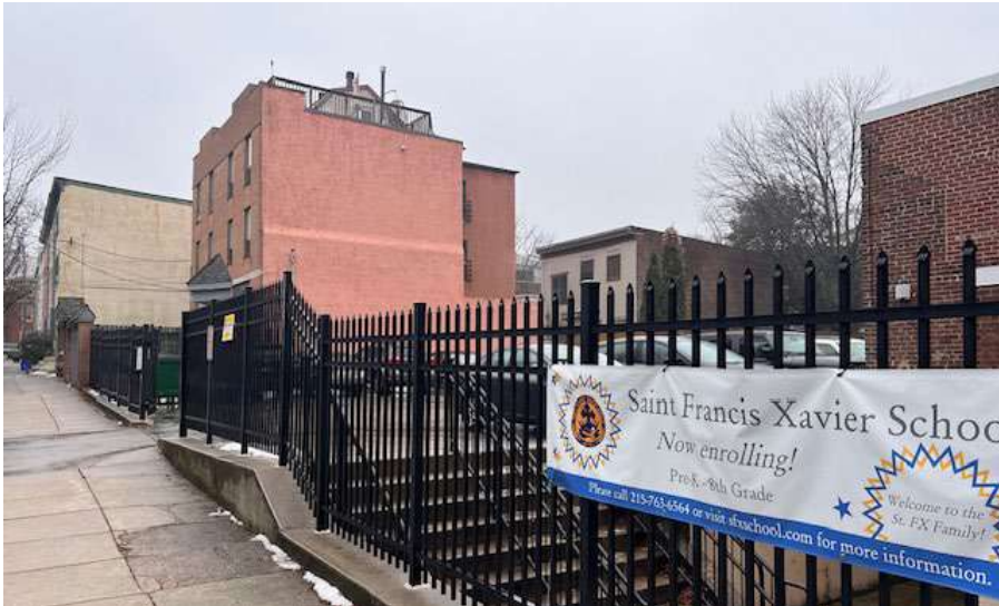
SITE PHOTOS, ADJACENT CONTEXT FROM WALLACE ST
