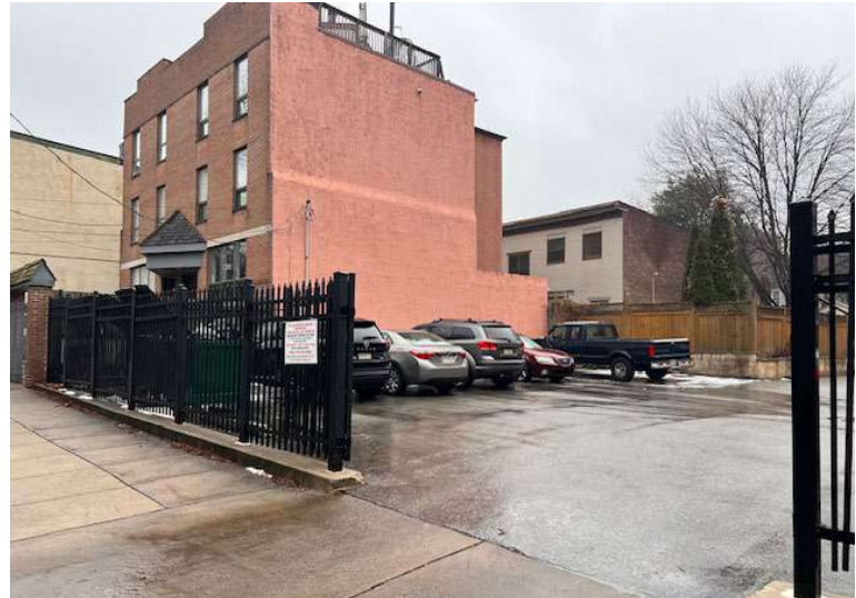
SITE PHOTOS, ADJACENT CONTEXT FROM WALLACE ST
