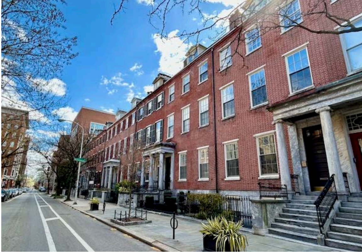
Photograph 9: Looking southeast along the 900 block of Spruce Street at Portico Row.
