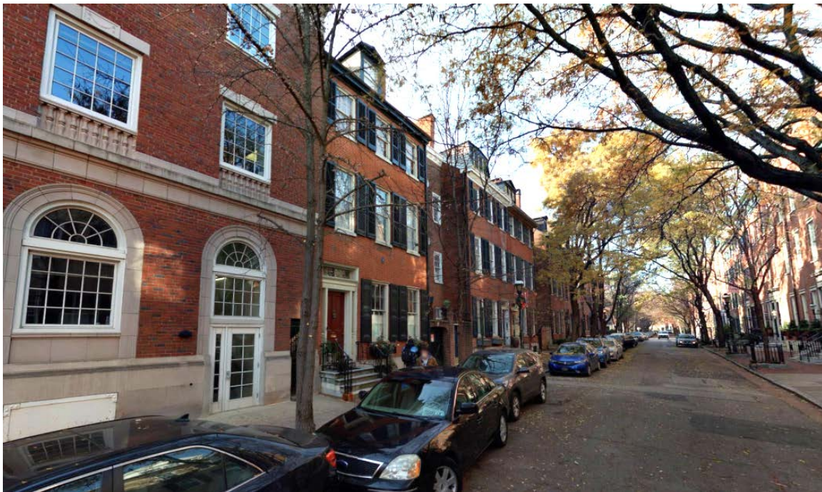
Photograph 18: Looking southwest along the 900 block of Clinton Street. Cyclomedia, December 2021.
