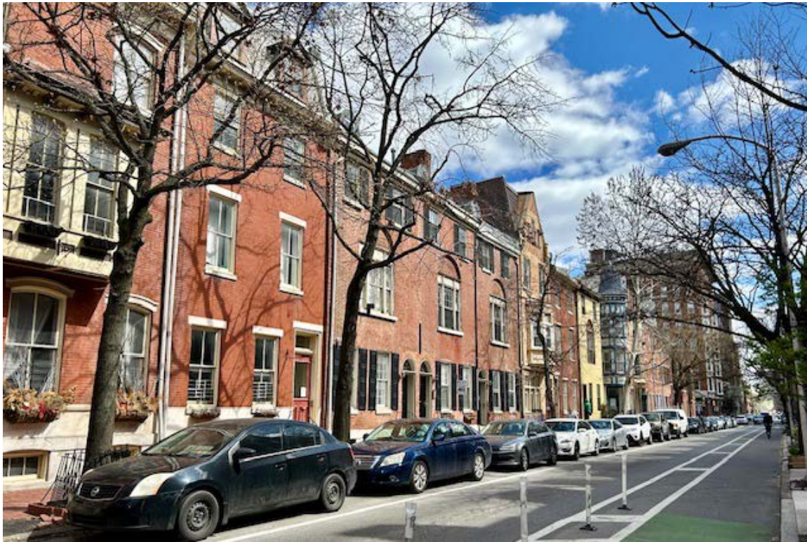
Photograph 8: Looking northeast along the 900 block of Spruce Street.
