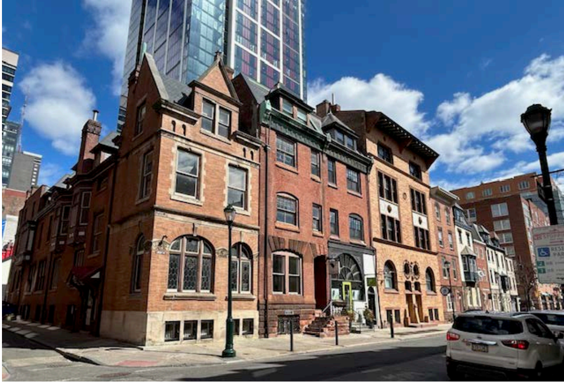
Photograph 3: Looking northeast from Camac and Locust Streets along the 1300 block of Locust Street.
