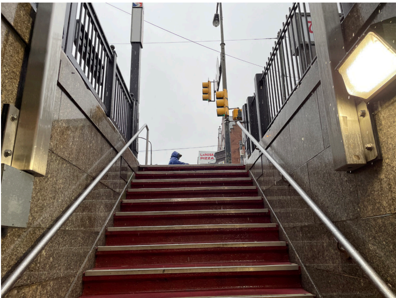
1 NORTHWEST CORNER STAIRWELL
