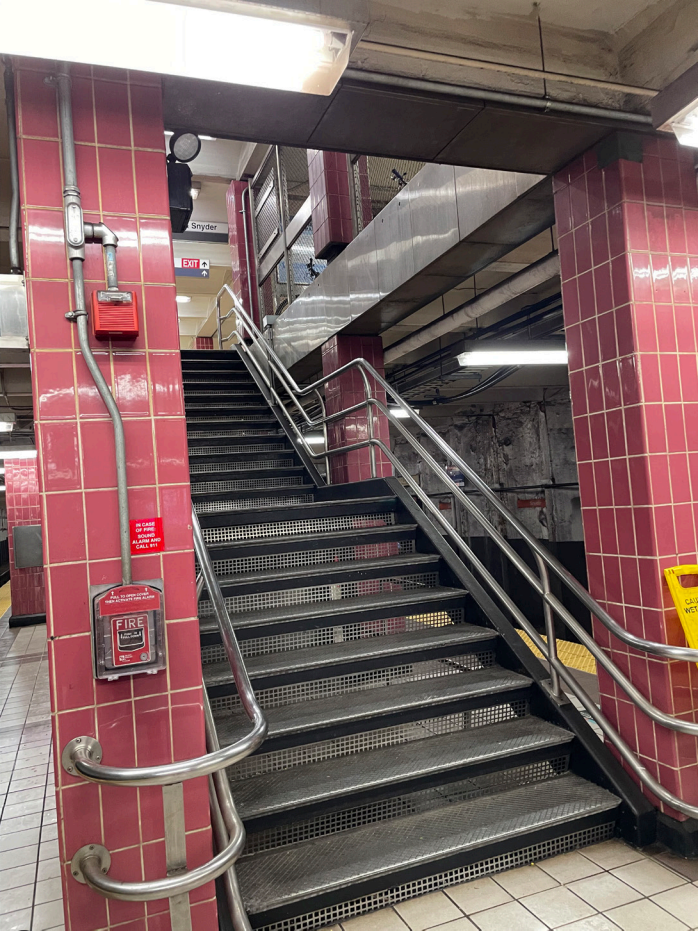
3 PLATFORM TO MEZZANINE STAIR - FINISH REPLACE-
