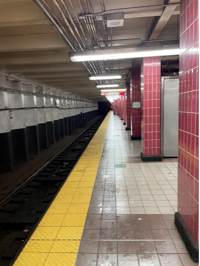
2 PLATFORM MID-AREA - FINISH REPLACEMENT
