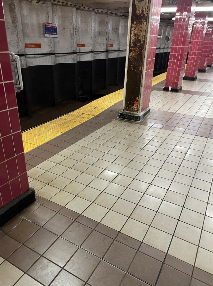
4 PLATFORM GENERAL - FINISH REPLACEMENT
