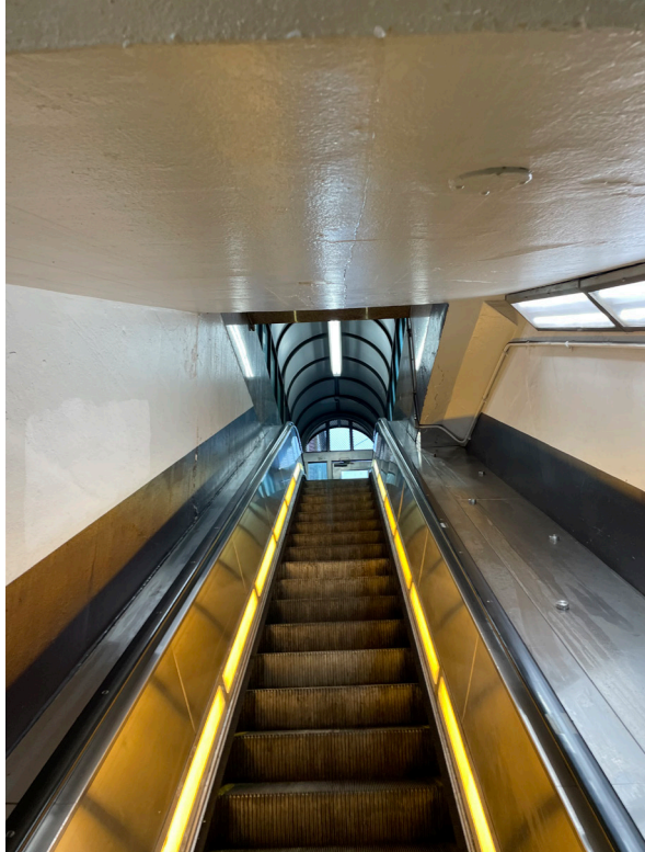
4 SOUTHWEST ESCALATOR (TO BE DEMOLISHED)
