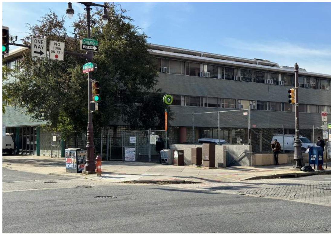
1 PERSPECTIVE OF EXISTING NW STAIR LOOKING SW A-27
