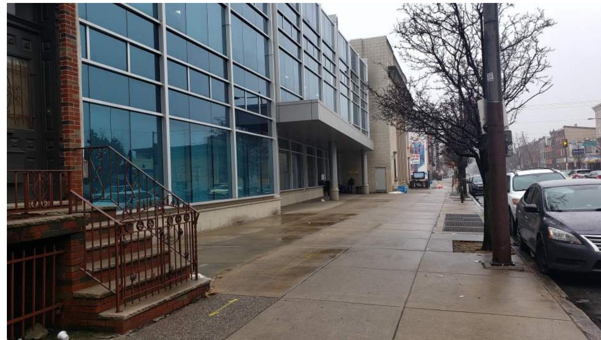
3 PERSPECTIVE OF EXISTING STOOP LOOKING SOUTH A-27
