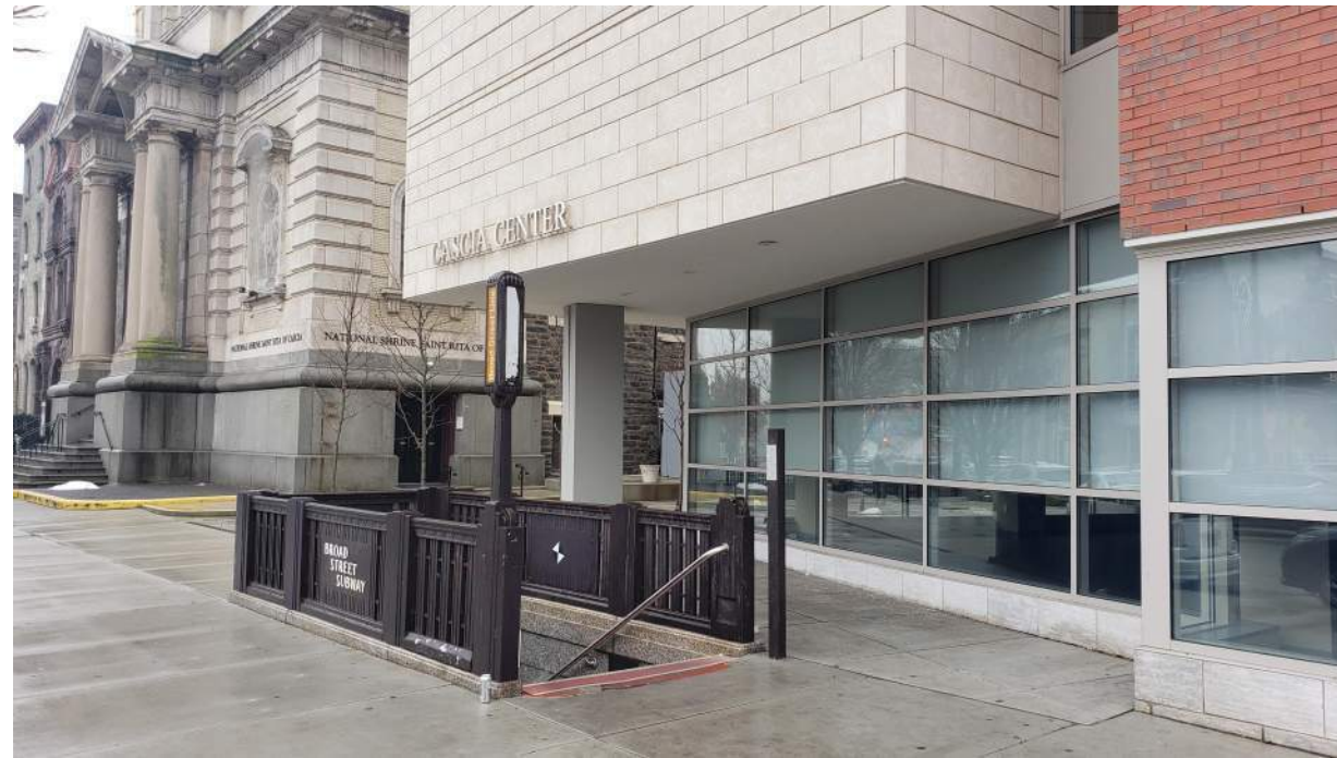
1 PERSPECTIVE OF EXISTING NW STAIR LOOKING SW A-27
