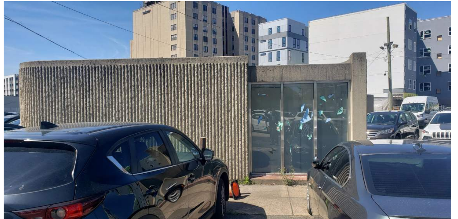
VIEW OF EAST EXISTING EGRESS STAIR HEADHOUSE LOOKING SOUTHWEST
