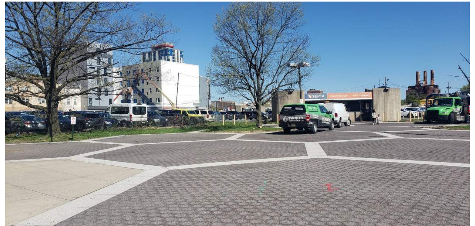
VIEW OF HEADHOUSE & PLAZA LOOKING NORTHWEST
