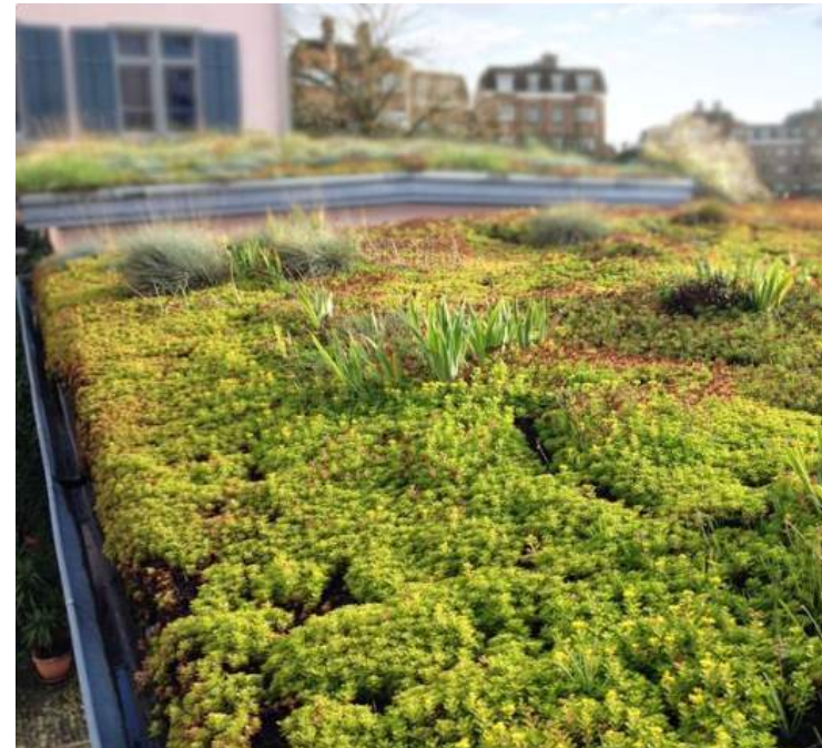
GREEN ROOF EXTENSIVE
