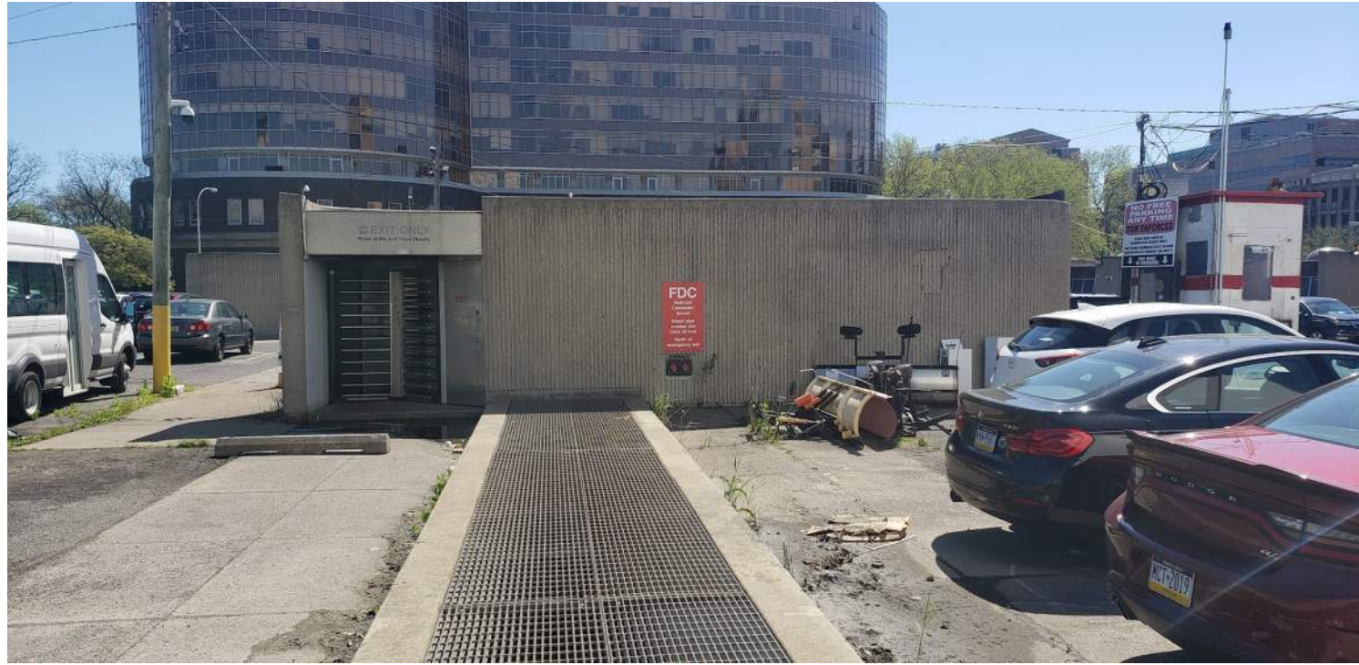
VIEW OF WEST EXISTING EGRESS STAIR HEADHOUSE LOOKING EAST
