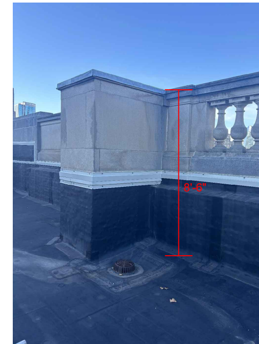
MEASUREMENT TAKEN AT WEST FACADE ROOF BALUSTRADE
