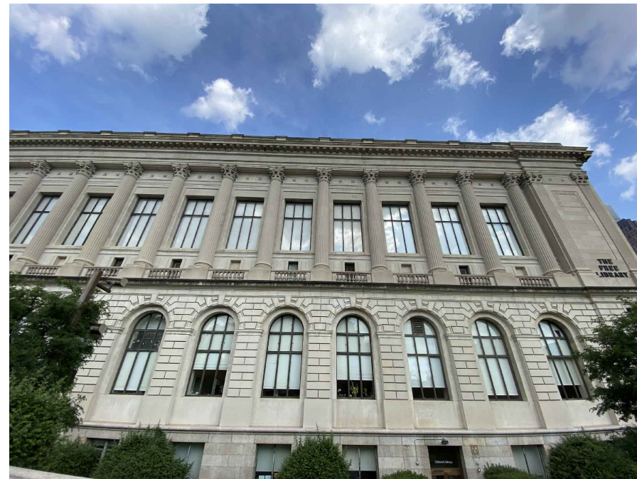
VIEW FROM SIDEWALK AT 20TH STREET
