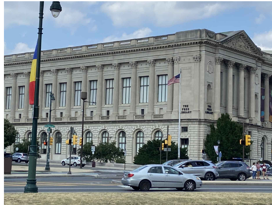
250 FT FROM SITE, VIEW FROM SOUTH SIDE OF BENJAMIN FRANKLIN PARKWAY
