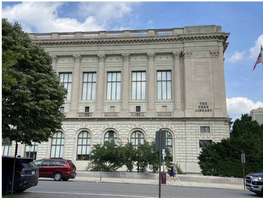
50 FT FROM BUILDING, VIEW FROM 20TH STREET
