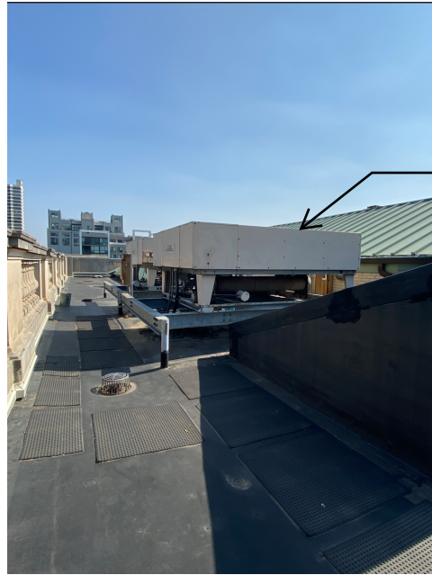
VIEW FROM UPPER ROOF, FACING NORTH.
