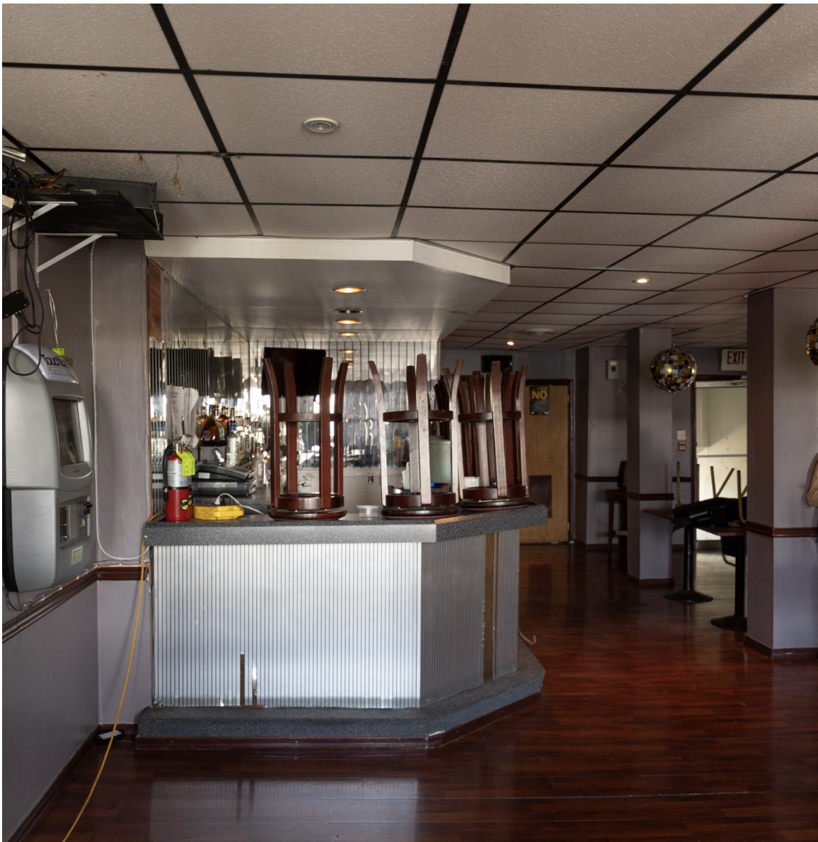
Figure 6.17: The third-story bar installed by Mr. Adams in the 1990s.
