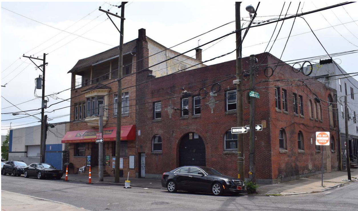
Figure 6.6: The north and west elevations of New Barber's Hall
