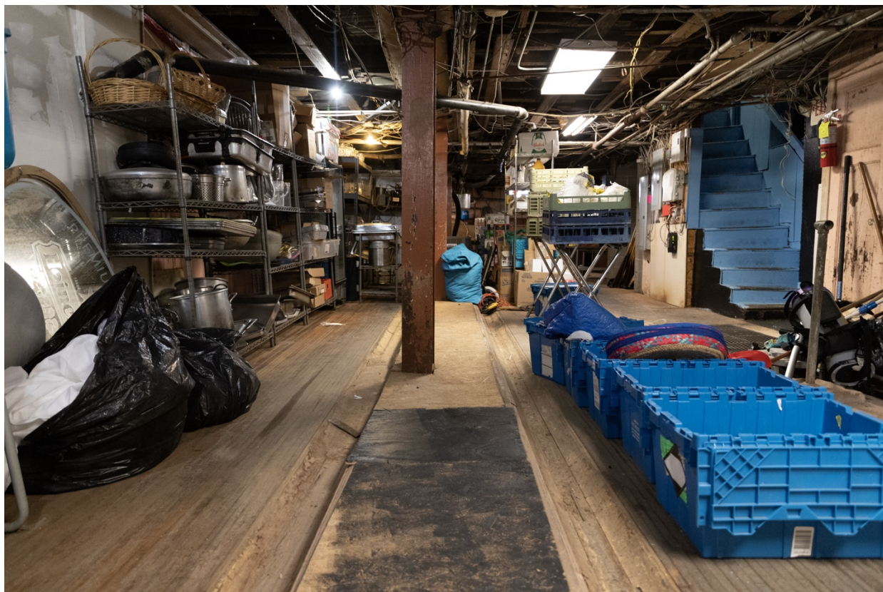
Figure 6.21: There are two largely-intact bowling lanes in the basement of 1402-04 West Oxford Street. Oriented strand board covers the uneven space between the two lanes, likely concealing additional surviving features from the bowling alley.
