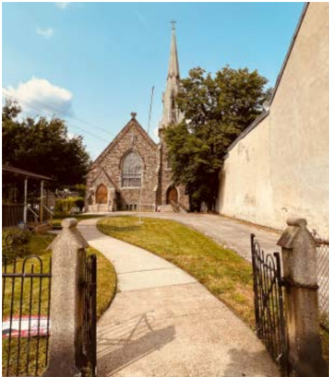
Figure 1: View of the building from Germantown Avenue.
