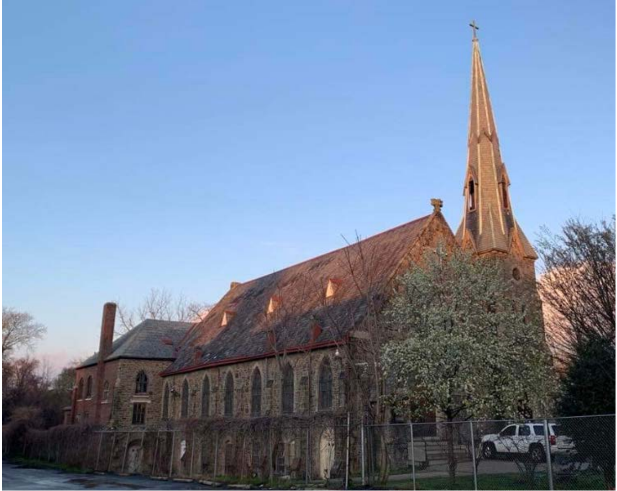
Figure 2: View of subject building from the West.
