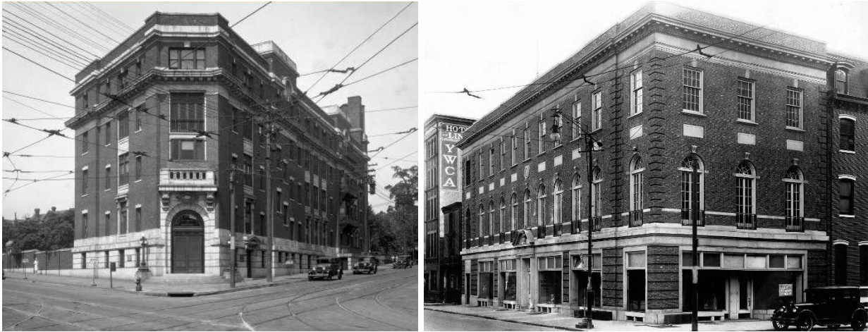
Figure 7 (left) – Rush Hospital, 33rd and Lancaster, 1931, extant (Philadelphia Department of Records). Figure 8 (right) – The Philadelphia Real Estate Board Building at 13th and Locust Streets in the 1920s, extant (Ballinger Collection, Athenaeum of Philadelphia).
