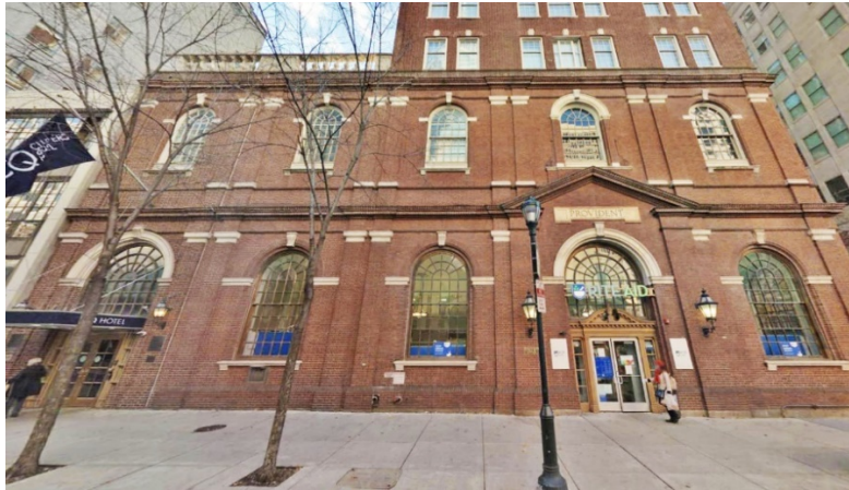
Photo 2 – North elevation, showing the first and second stories. From right to left, the first three bays consist of the original 1927-28 building, the fourth bay consists of the 1946 addition, and the fifth or leftmost bay consists of the 1987 addition.
