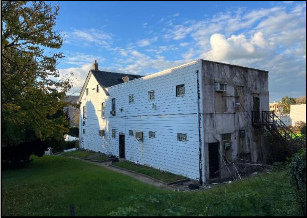
Figure 6. Looking northeast at the Douglas Political Club, showing the southwest and southeast elevations. Source: Oscar Beisert, 2023.
