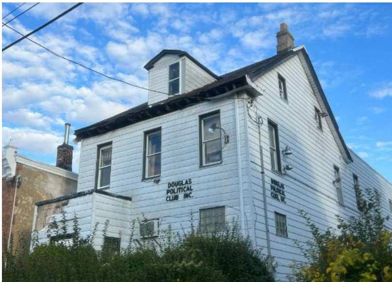
Figure 1: Front façade of subject building.
