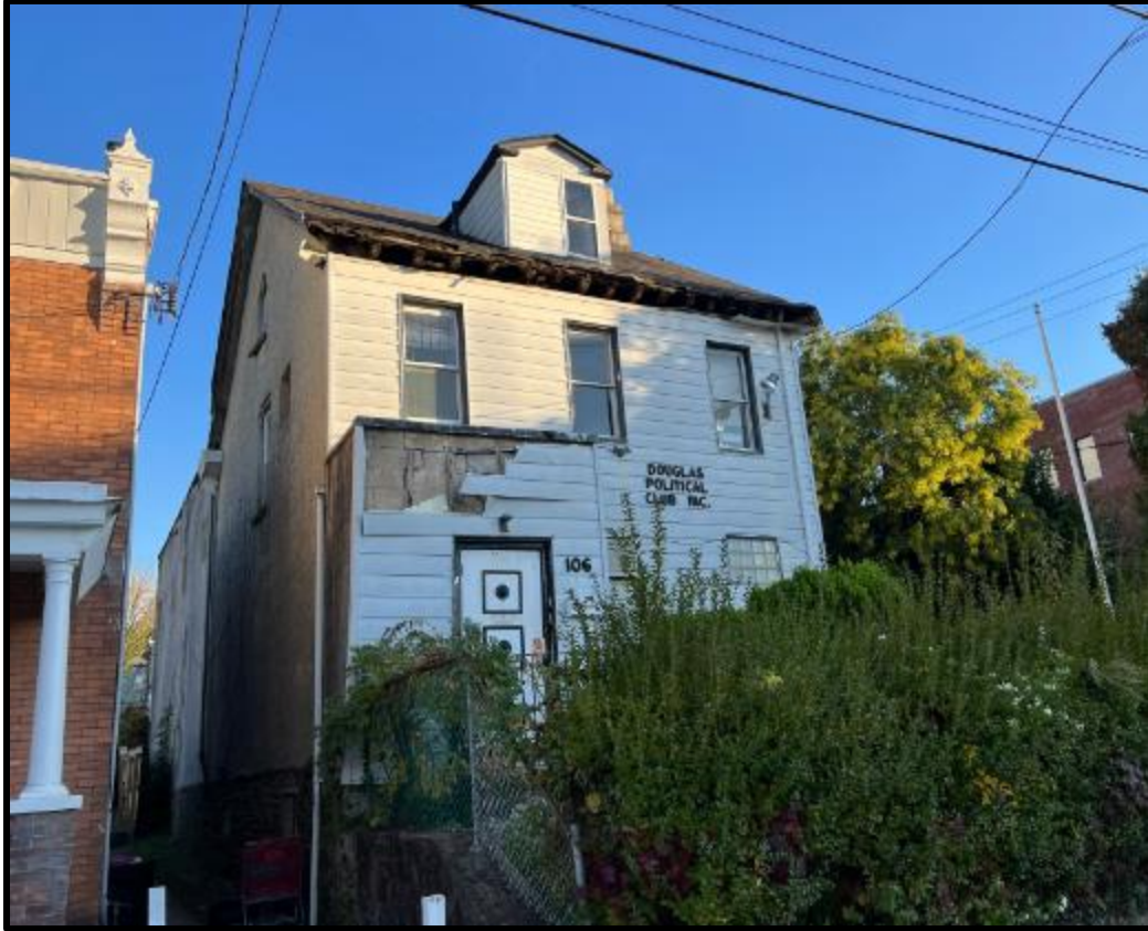
Figure 5. The Douglas Political Club, 106 E. Sharpnack Street, Side (Northeast) and Primary (Northwest) Elevations. Source: Oscar Beisert, 2023.
