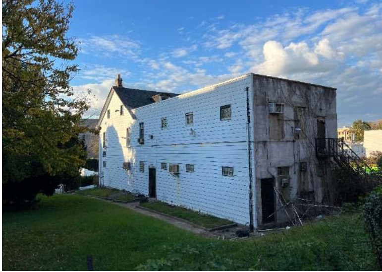
Figure 2: View of the rear of subject building.
