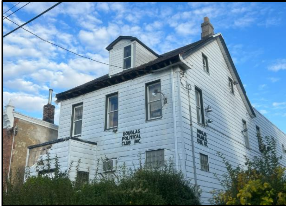
Figure 3. The Douglas Political Club, 106 E. Sharpnack Street, Primary (Northwest) and Side (Southwest) Elevations. Source: Oscar Beisert, 2023.
