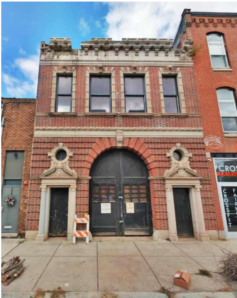
Figure 1: South elevation of the Engine 13 Firehouse, facing Parrish Street.
